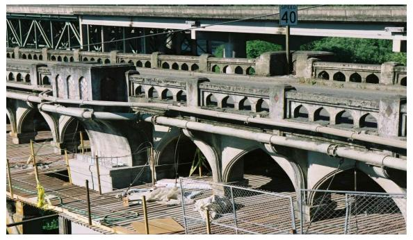
Figure D-3: North Umpqua River (Old Winchester) Bridge, Oregon, showing the original bridge rail and pedestrian refuge.
