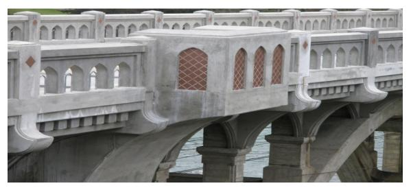
Figure D-4: North Umpqua River (Old Winchester) Bridge, showing new stealth rails with arch hoops and pedestrian refuge.
