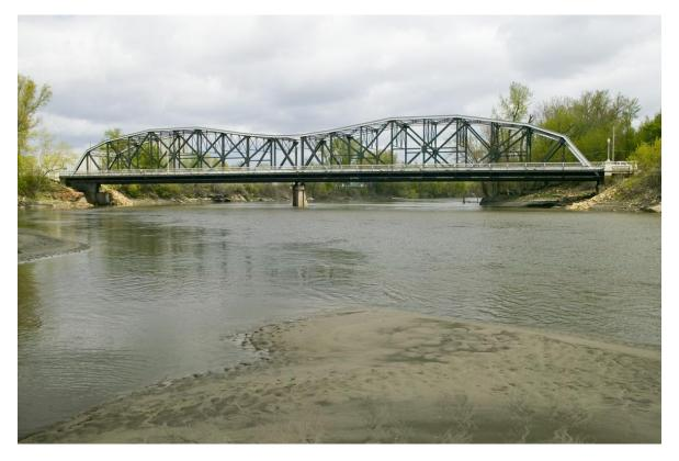
Figure D-14: Broadway Bridge, Number 4930, Minnesota River, Steel Through-Truss, 1931, MNDOT
