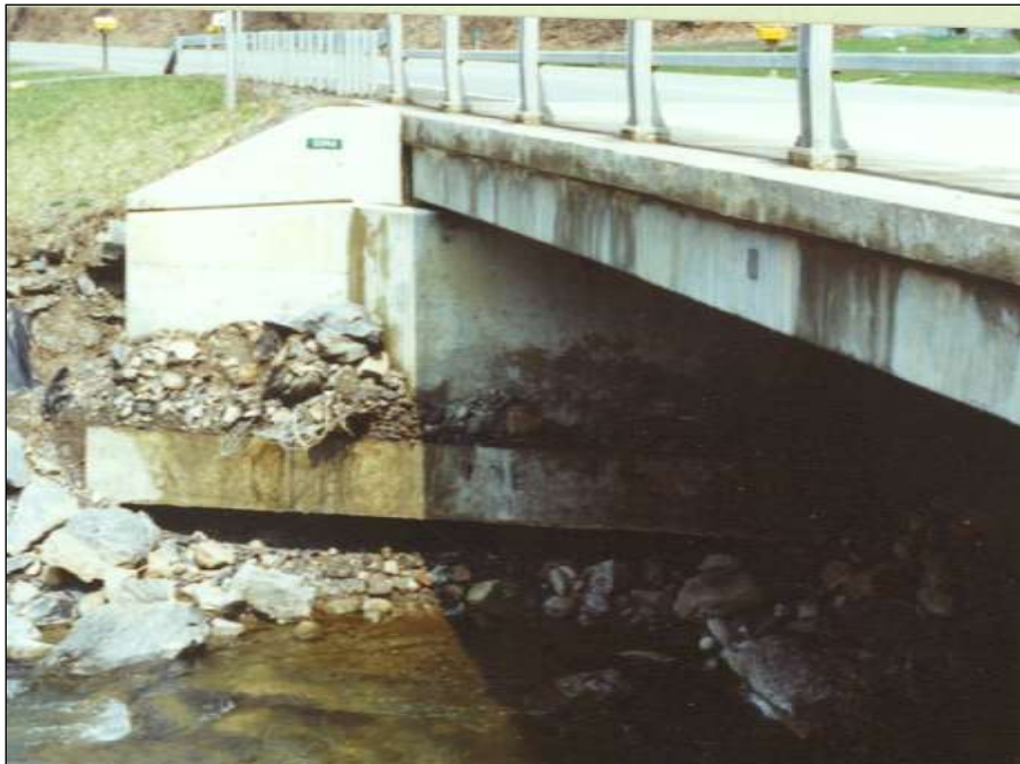
Figure 1-2. A wing-wall abutment with earthfill approach embankment
