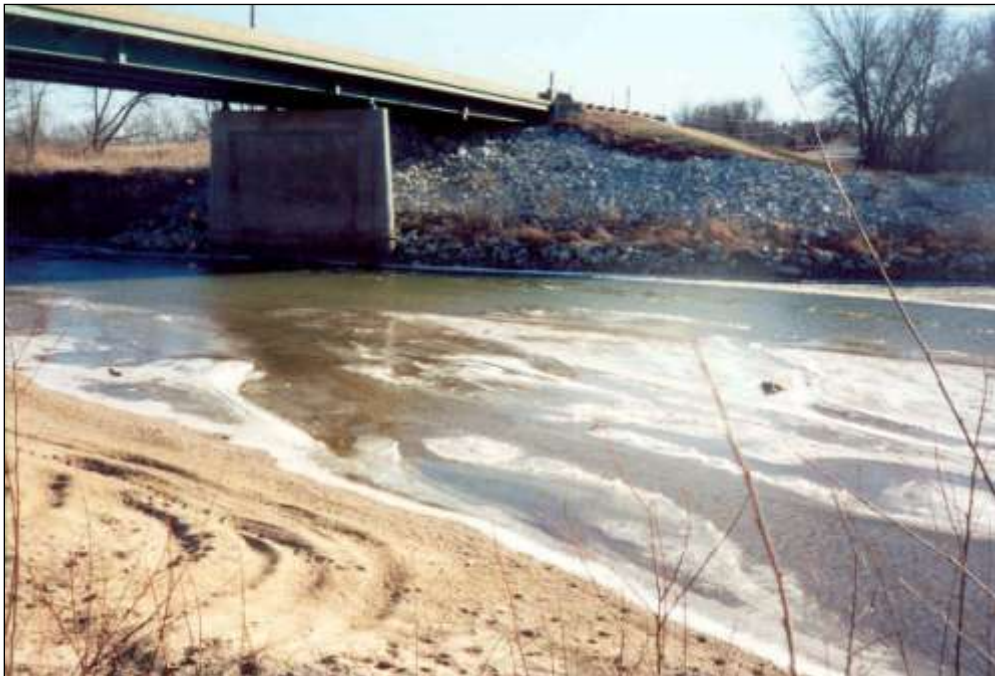
Figure 2-6. A spill-through abutment with a pier in close proximity; approximate layout proportions of L/B_f = 1.0 ; B_f/0.5B \approx 0.7 , and L/W \approx 1.0 , in which W = abutment top width
