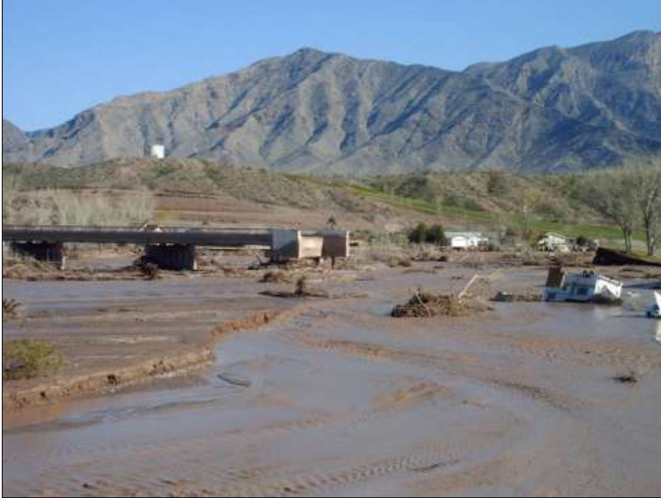
Figure 3-8. Scour Condition C at a spill-through abutment
