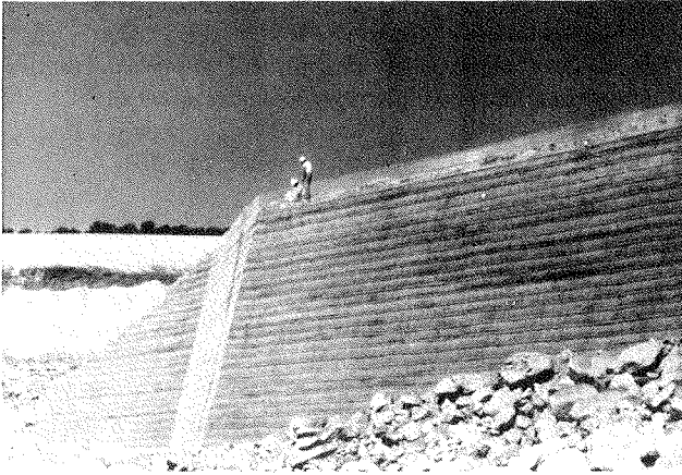
Figure B-6. Photograph of Chevron double wall under construction.
