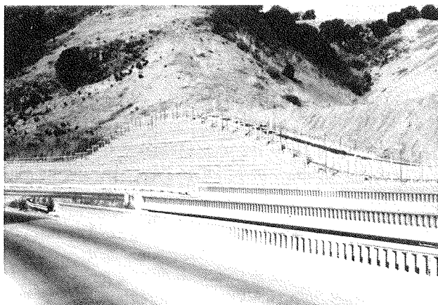
Figure B-4. Photograph of Welded Wire Wall in highway applications.
