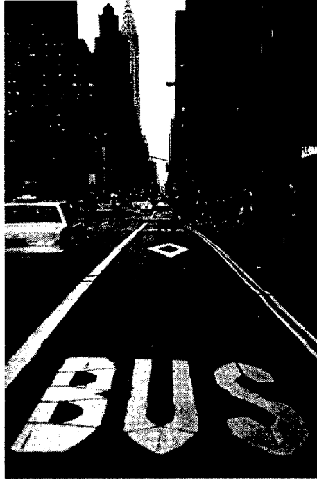
Figure 8-31. Example of Diamond Pavement Marking with Arterial Street HOV Lane
