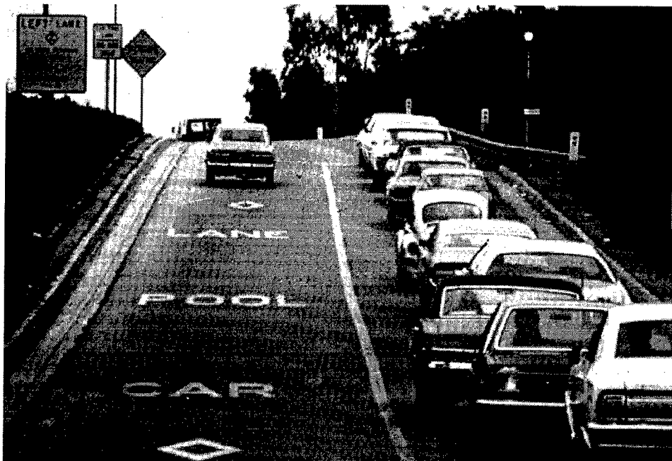
Figure 2-12. HOV Bypass Lane at Metered Freeway Entrance Ramp in Southern California
