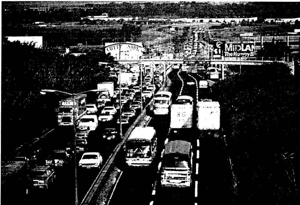
Figure 5-10. Contraflow Lane on I-495 in Union City, New Jersey
