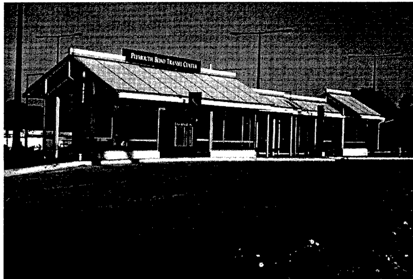
Figure 9-12. Off-line Centers on the I-394 HOV Lanes
