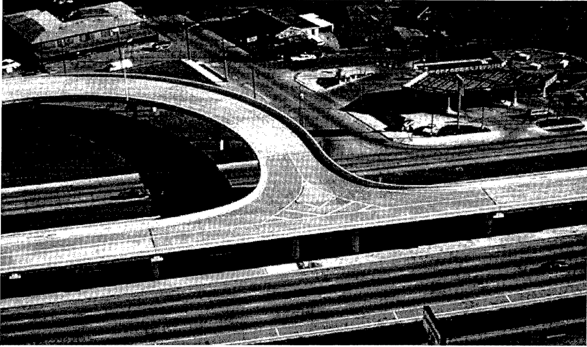
Figure 2-15. T-Ramp in Houston
