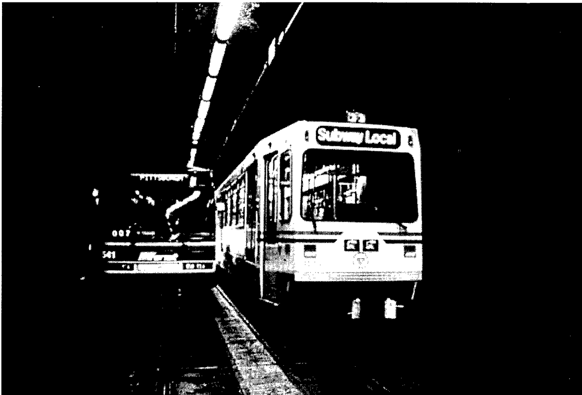
Figure 9-20. Bus and LRT Vehicle in Mount Washington Tunnel
