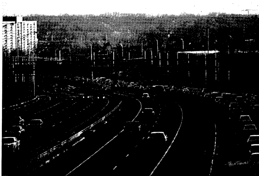
Figure 2-7. Exclusive Two-Lane Reversible HOV Facility— I-395 (Shirley Highway) HOV Lanes in Northern Virginia/Washington, D.C.
