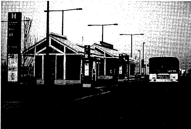
Figure 5-21. Examples of Supporting Facilities Frequently Found with HOV Lanes
