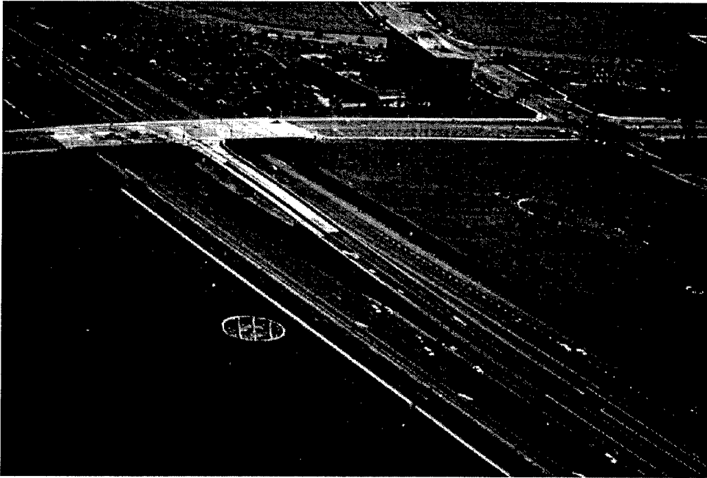
Figure 5-18. Drop Ramp in Orange County, California
