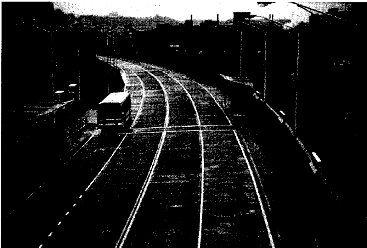
Figure 2-25. On-line Station on the Pittsburgh Busway
