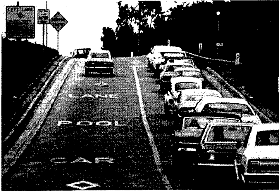
Figure 5-12. HOV Bypass Lane at Metered Freeway Entrance Ramp in Southern California
