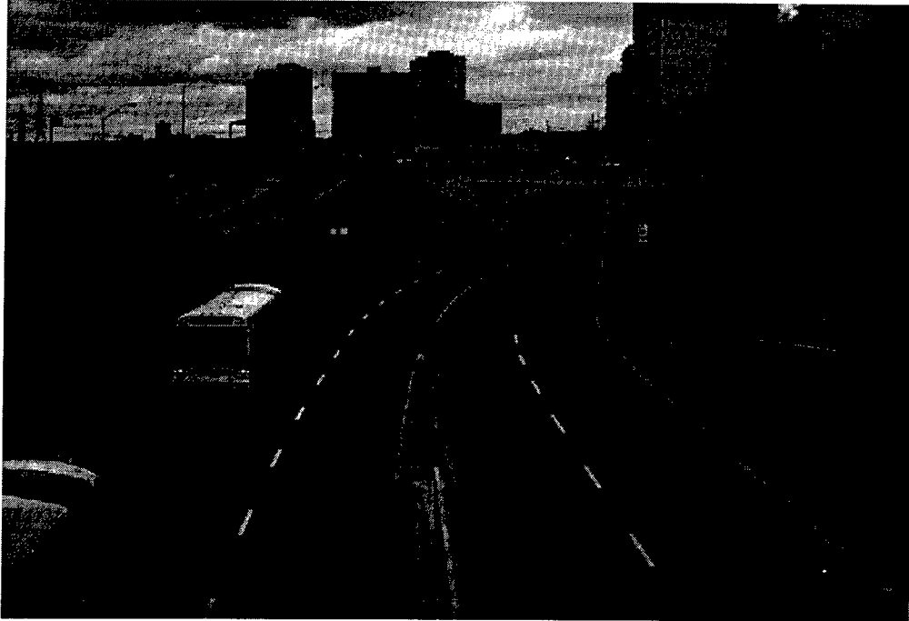
Figure 2-4. Bus-only Facility in Separate Right-of-Way—Ottawa Transitway
