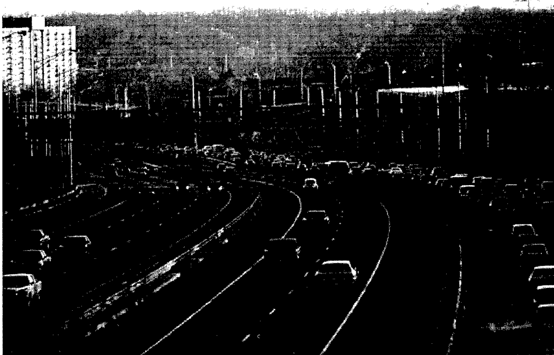
Figure 5-6. I-395 (Shirley Highway) HOV Lanes in Northern Virginia/Washington, D.C.
