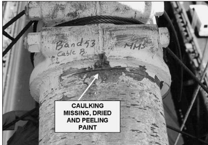
Figure 2.3.1.2.2-1 Damaged caulking and paint at cable band.
