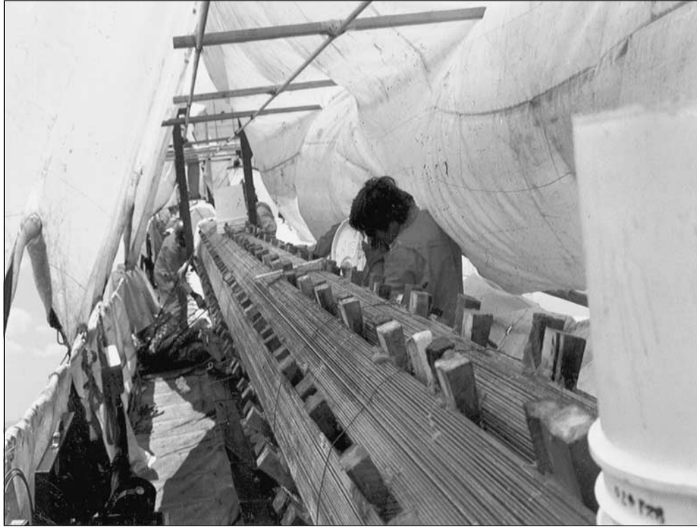
Figure 2.4.8.1-1. Inspection during cable rehabilitation.
