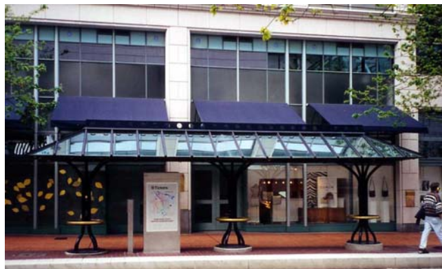
Figure 10.6 A Transit Shelter Located Curbside
