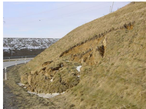
Figure 1: Slope slumping failure along roadway (Wikipedia)
