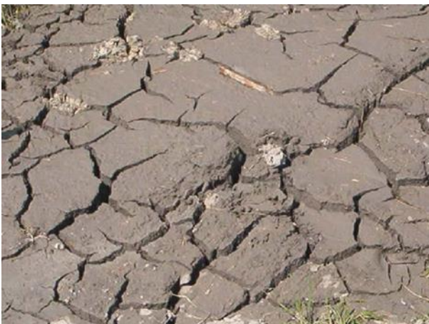
Figure 2: Desiccation cracking upon drying indicates likely presence of expansive soil conditions ( http://www.geology.ar.gov/images/mudcracks.jpg )
