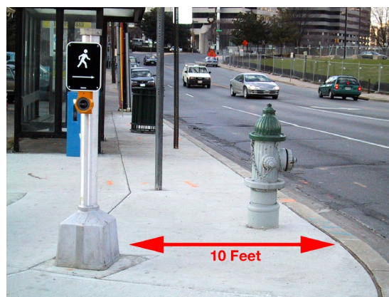
Figure 11. Pushbuttons should be a maximum of 10 ft from the curb line.
