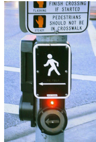
Figure 7. APS with actuation indicator light illuminated. Light remains illuminated until the call is serviced.
