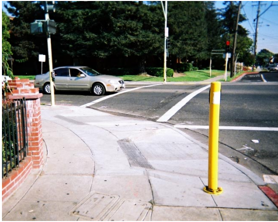
Figure 14. APS are positioned appropriately at this intersection by the addition of a stub pole for one crosswalk. The stub pole holding the APS for the crosswalk at right is simply bolted in. The other APS is mounted on the pole that supports the pedhead.
