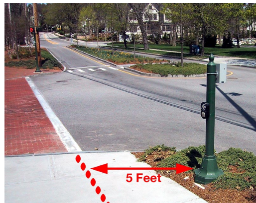
Figure 10. Pushbuttons should be a maximum of 5 ft from the crosswalk line extended.
