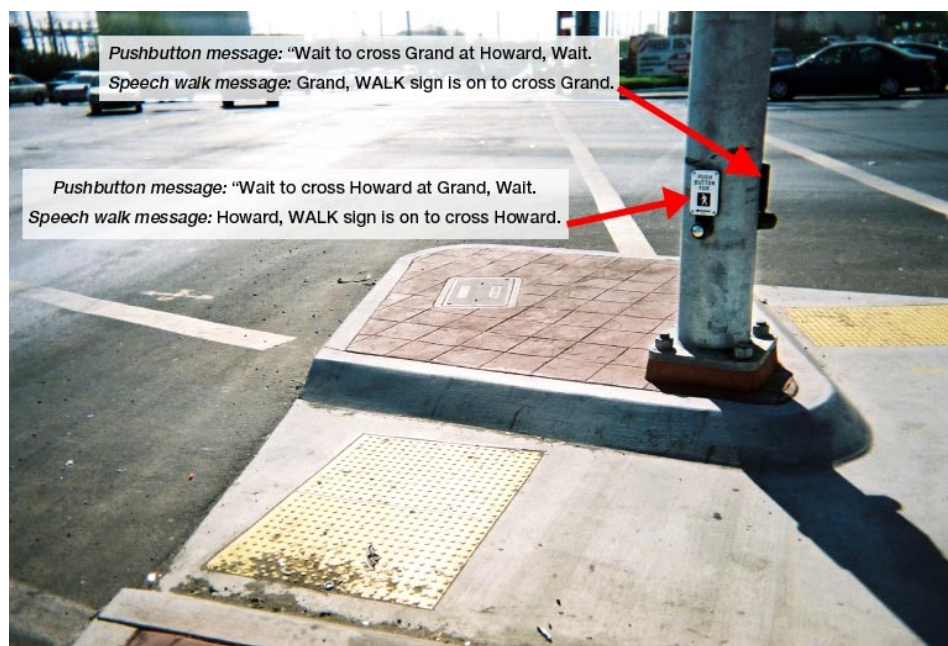
Figure 13. Speech walk messages and pushbutton information messages needed when two pushbuttons must be installed on the same pole. This should be last choice, if APS cannot be separated by 10 ft.
