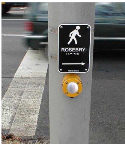
Figure 9. Braille label is located on the face of the APS device, just below the street name in large print.
