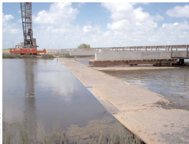
Figure 3 While barges are used typically to provide construction equipment access in open water situations, this Dura-Base composite mat system was used to provide worker access at the Cavasso Creek bridge project in Aransas County, TX.
