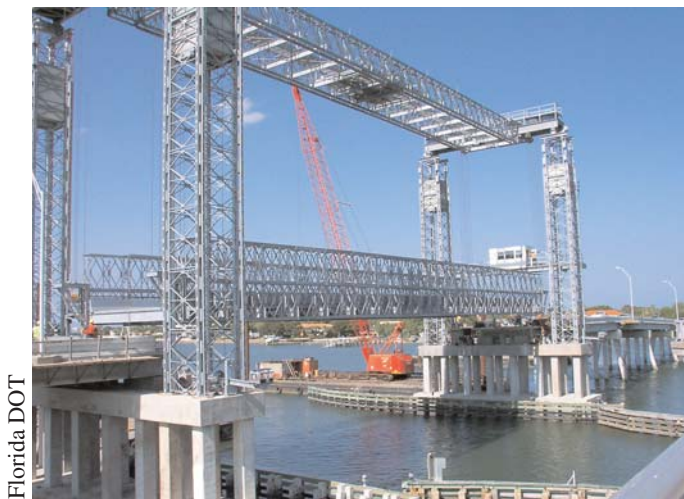
Figure 7 Acrow temporary vertical lift span, Bridge of Lions, St. Augustine, FL.
