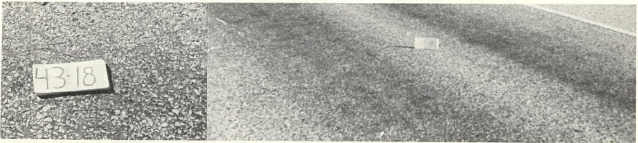
A chip seal in which the asphalt is filling the surface between the seal aggregate but has not covered the aggregate. (Rating 3.0)
