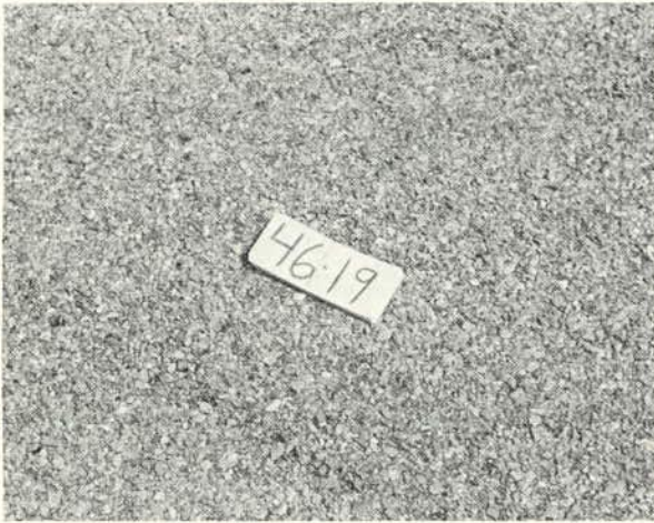
A chip seal with 100 percent of the surface covered with seal aggregate. (Rating 5.0)
