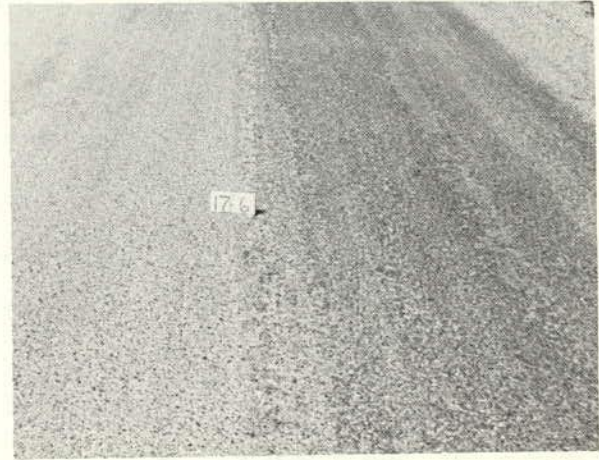
A chip seal with between 10 and 50 percent of the seal coat aggregate worn off between the wheelpath on the lane to the right. (Rating 3.0)
