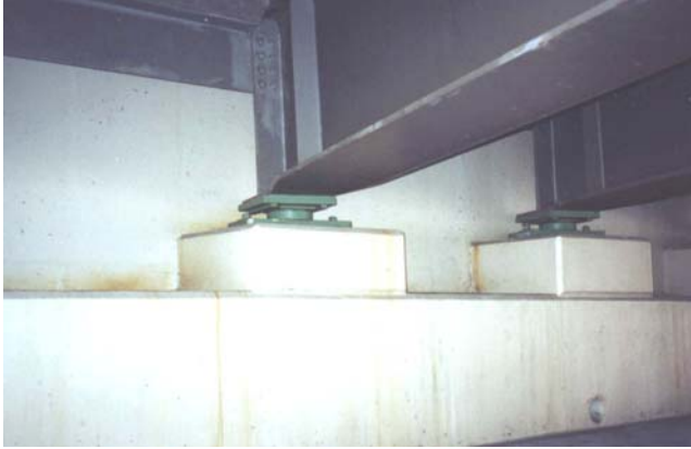
FIGURE 37 Seats and beam-ends under watertight compression seal installed in 1986.
