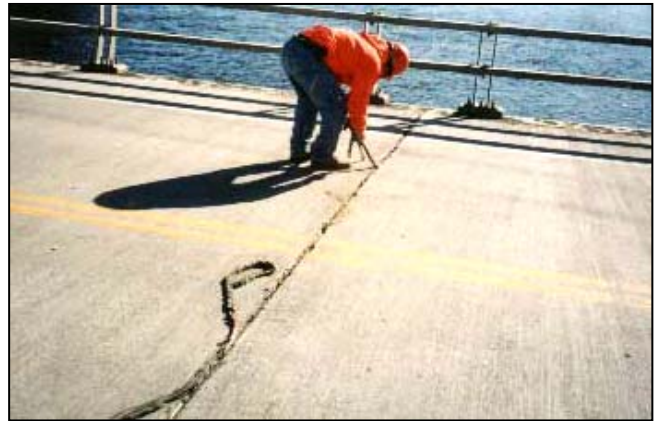
FIGURE 22 Removing failed poured-in-place sealant.
