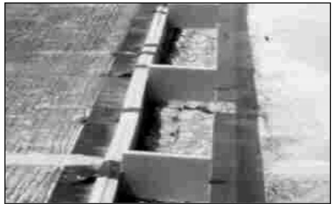
FIGURE 40 Blockout for joint replacement.
