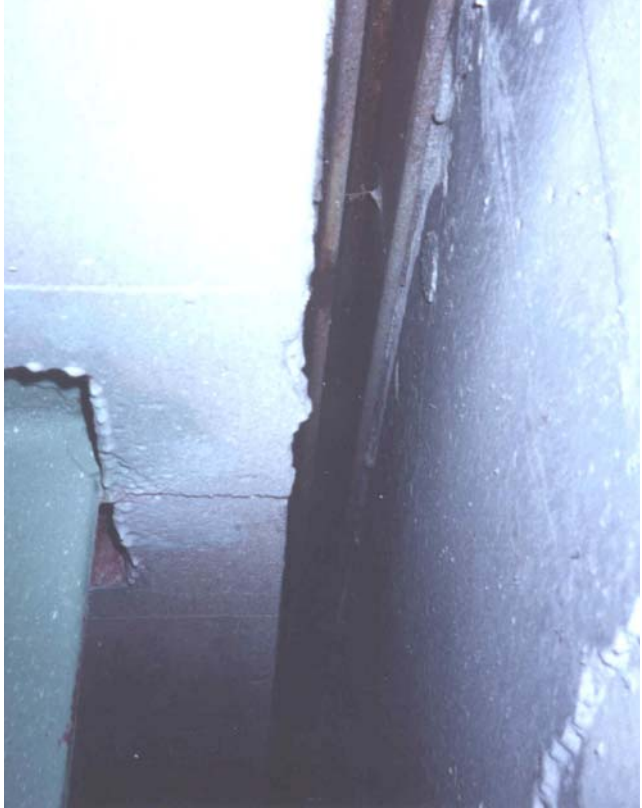
FIGURE 39 Under watertight strip seal, New York State Thruway.
