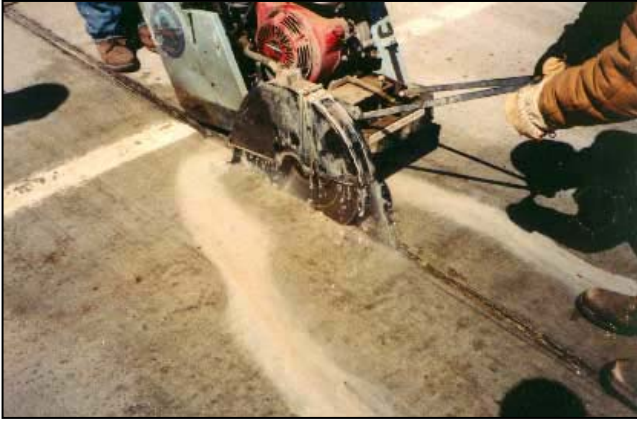
FIGURE 43 Saw cutting a joint opening.
