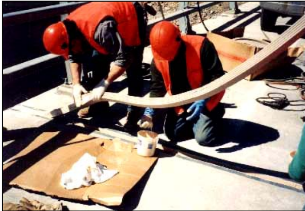
FIGURE 27 Placement of closed cell compression seal.
