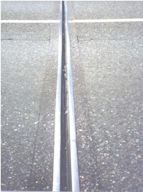
FIGURE 38 Top of watertight strip seal, New York State Thruway.
