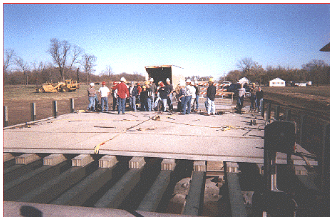
FIGURE 44 FRP deck panels made in a tongue and groove design for easier installation.
