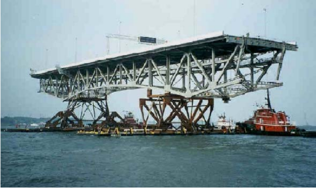
FIGURE 13 George P. Coleman Bridge. (Source: www.aashtotig.org ; courtesy: Virginia DOT.)
