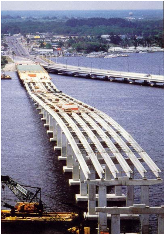
FIGURE 40 View of prefabricated substructure and girders of Edison Bridge.
