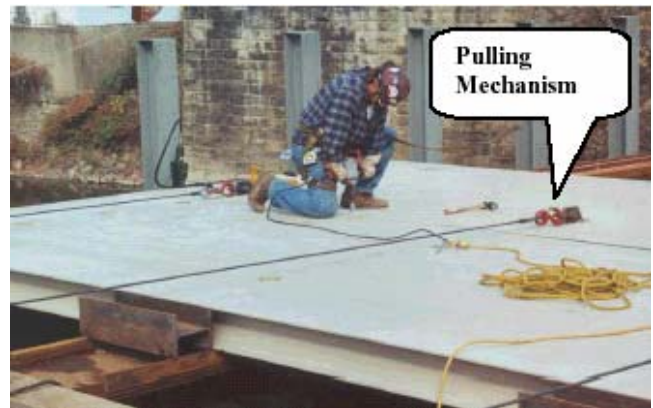
FIGURE 51 Pulling mechanism of modules. [Source: Shekar et al. (34).]
