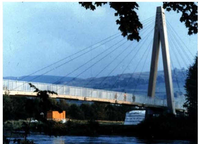
FIGURE 1 Aberfeldy footbridge over the River Tay in Scotland. (Source: http://www-civ.eng.cam.ac.uk/isegroup/uklocate.htm .)
