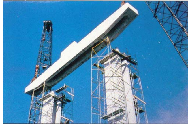
FIGURE 41 Installation of prefabricated bent cap in Edison Bridge.
