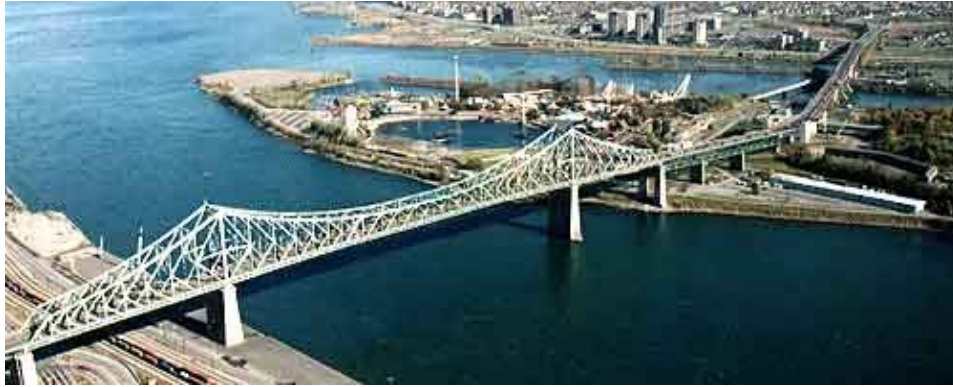
FIGURE 42 Jacques-Cartier Bridge. (Source: www.pjcci.ca .)
