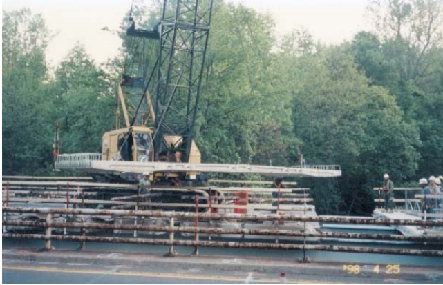
FIGURE 11 Dead Run and Turkey Run bridges. (Source: www.aashtotig.org ; courtesy: FHWA.)
