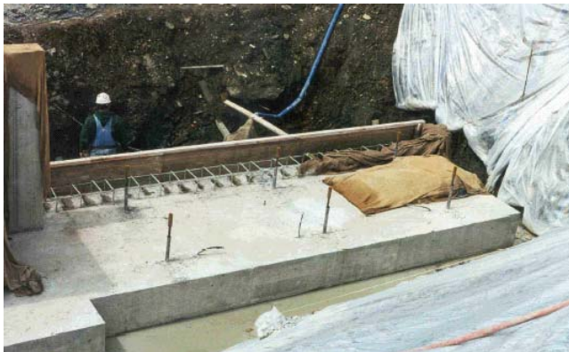
FIGURE 35 Cast-in-place footings with projecting dowels. [Source: Scanlon et al. (26).]
