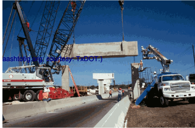
FIGURE 15 US-290 ramp E-3 bridge. (Source: www.aashtotig.org.)
