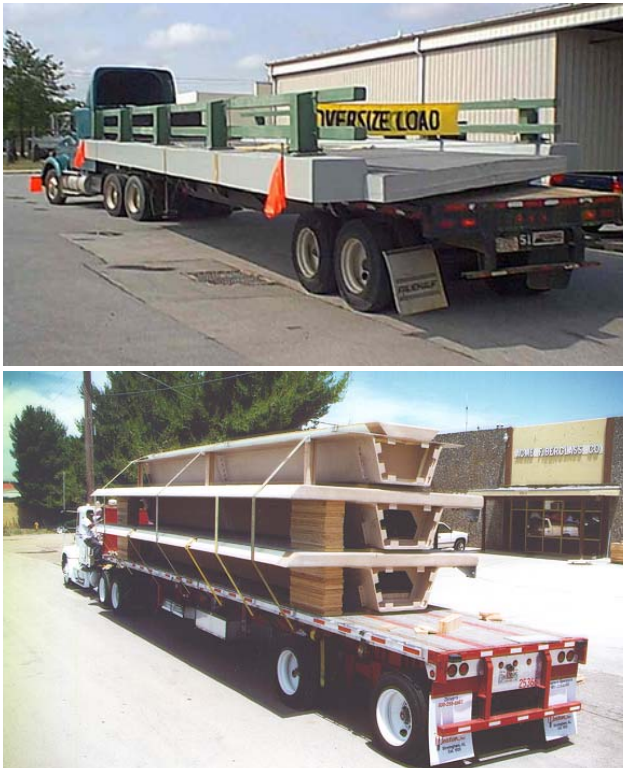
FIGURE 2 Fabrication and transportation of FRP bridge segments.
