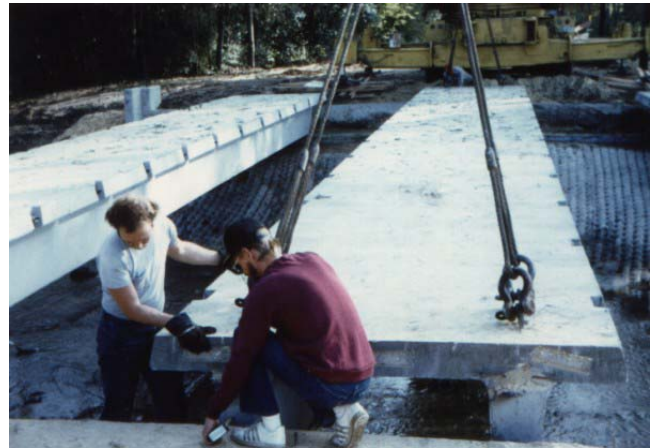
FIGURE 33 Construction of transversely posttensioned double-tees bridges.
