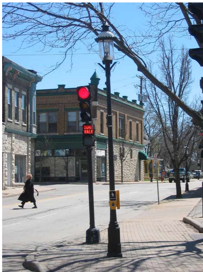
Figure 5-3. APS mounted on lamp post.
