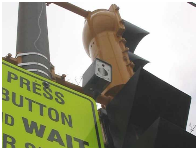
Figure 5-2. APS overhead speaker mounted on signal head support arm.
