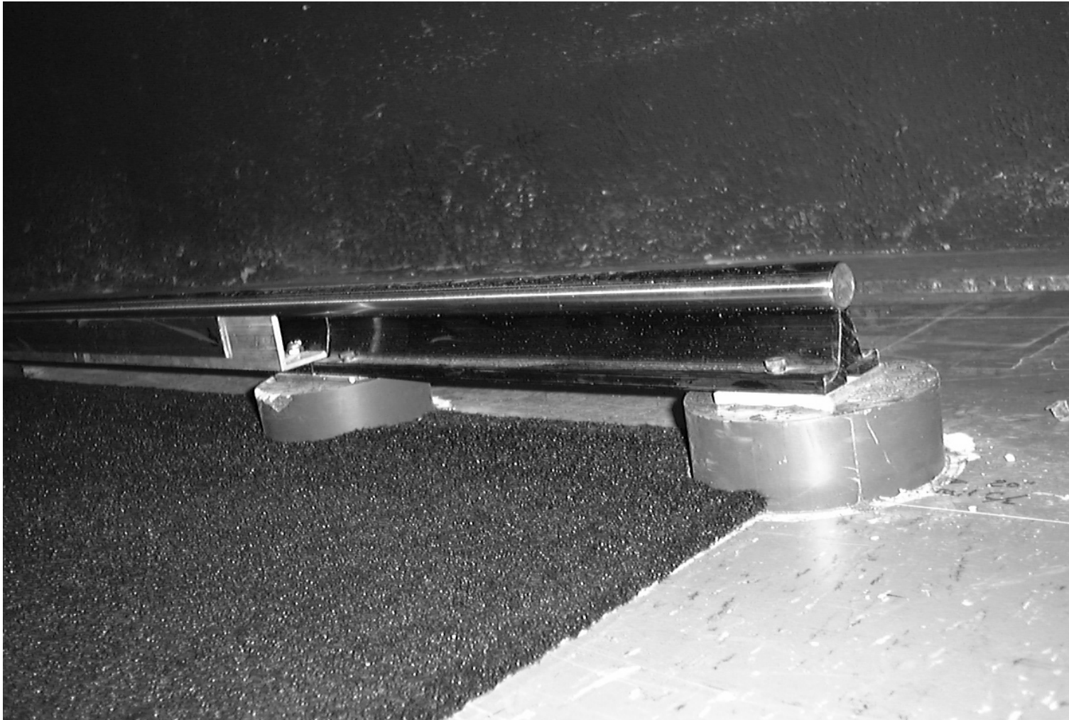
Figure 22 – Shown is a section of the rail system.
