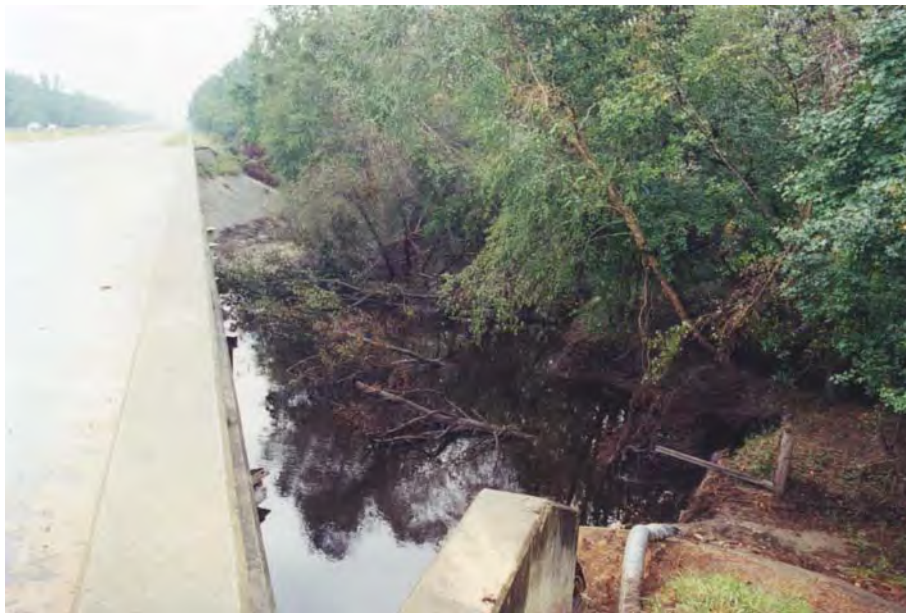
Figure 6. Looking downstream from the east bound bridge deck during low-flow.
