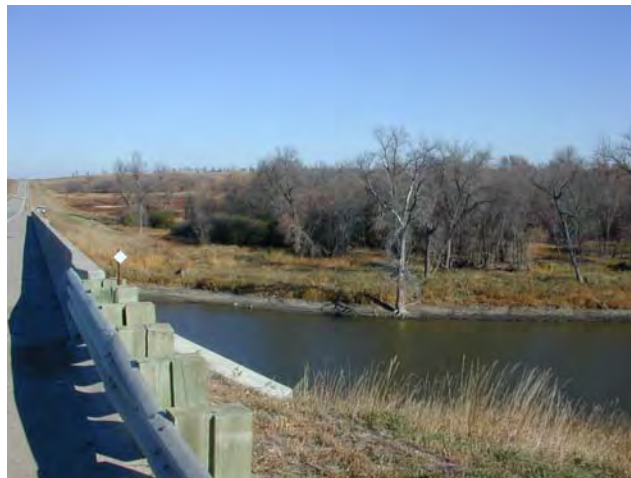
Figure 16. Post-flood conditions, looking at downstream left floodplain from S.R. 37 bridge.
