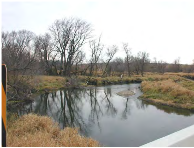
Figure 5. Looking downstream from County Route 22 bridge deck during low flow.
