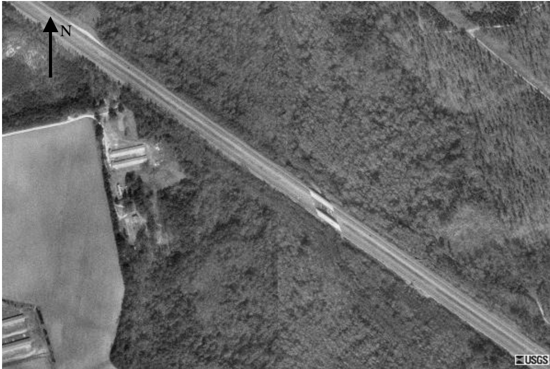
Figure 3. – Aerial photo of the U.S. 70 crossing over Bear Creek near LaGrange, NC.
