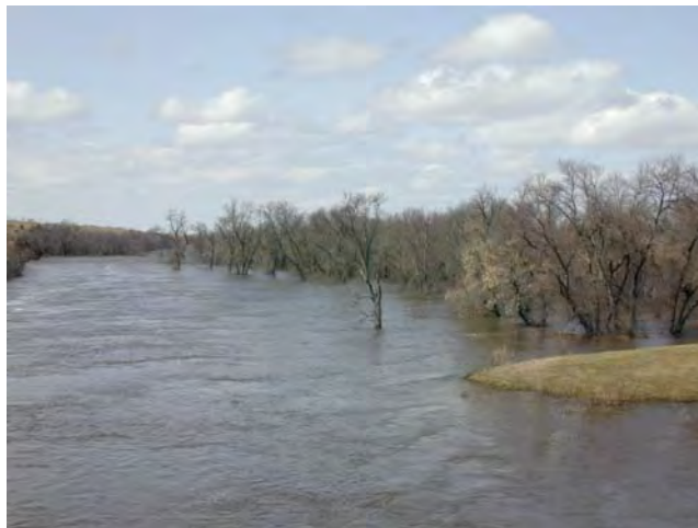
Figure 9. Looking upstream towards left floodplain from bridge deck
