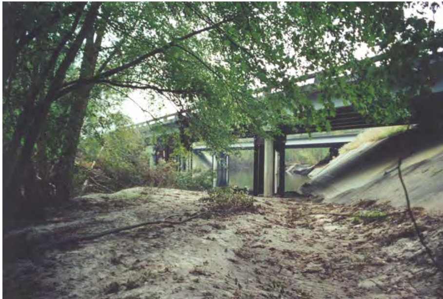
Figure 5. Looking upstream at the east bound bridge abutment during low-flow.
