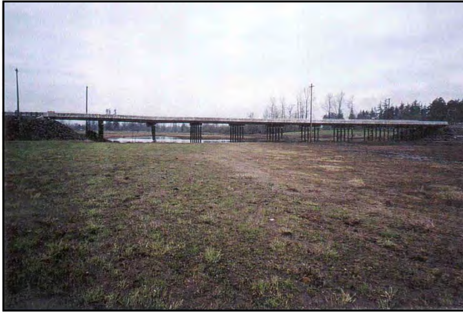
Figure 7. Looking downstream (north) to the Galvin Road overflow bridge.
