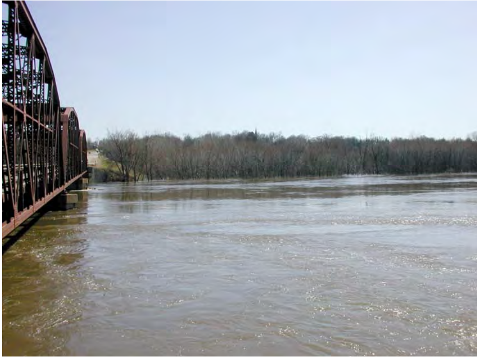
Figure 7. Looking at turbulent flow and eddy fence attributed to severe contraction along the upstream left abutment of the S.R. 25 bridge during the April, 2001 flood.
