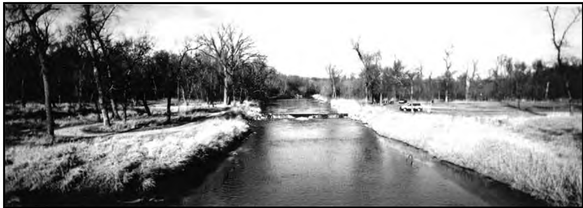
Figure 8. Looking upstream from U.S. 12 bridge deck at the small dam on the Pomme De Terre River during low-flow prior to the April, 1997 flood.
