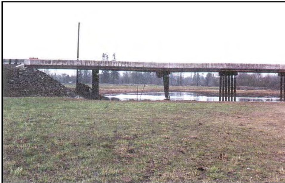
Figure 8. Looking downstream at piers 8, 9 (the pier that failed) and 10 following the February 1996 flood.
