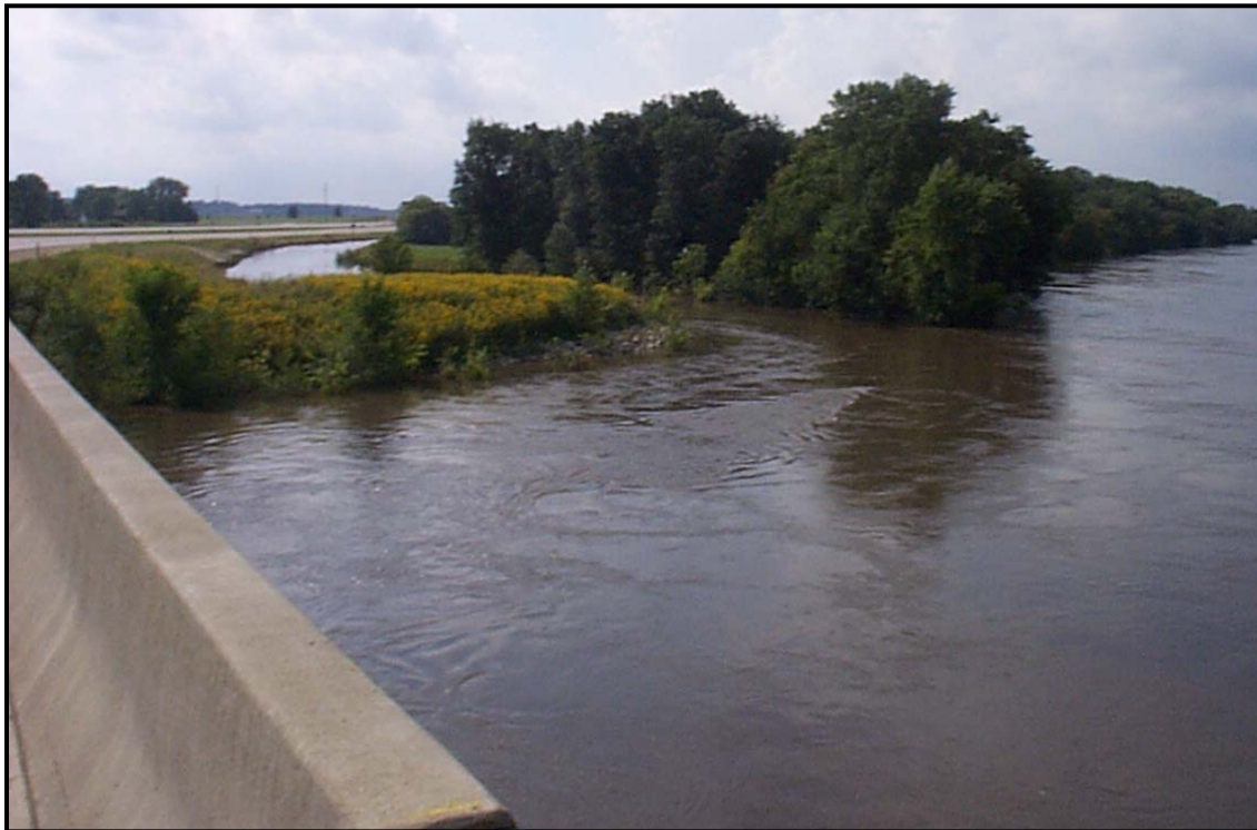
Figure 8. Looking upstream at right guide bank, floodplain and drainage ditch on 7/23/1999.
