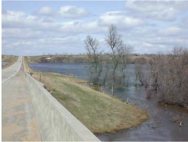
Figure 11. Looking at downstream left floodplain from bridge deck
