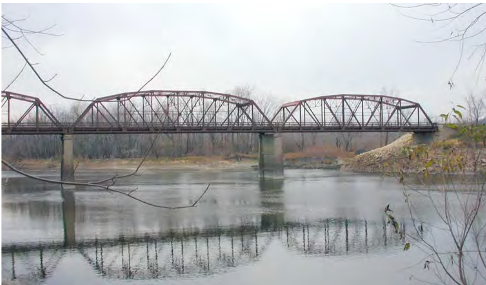
Figure 8. Looking upstream at S.R. 25 bridge and left abutment during low-flow.
