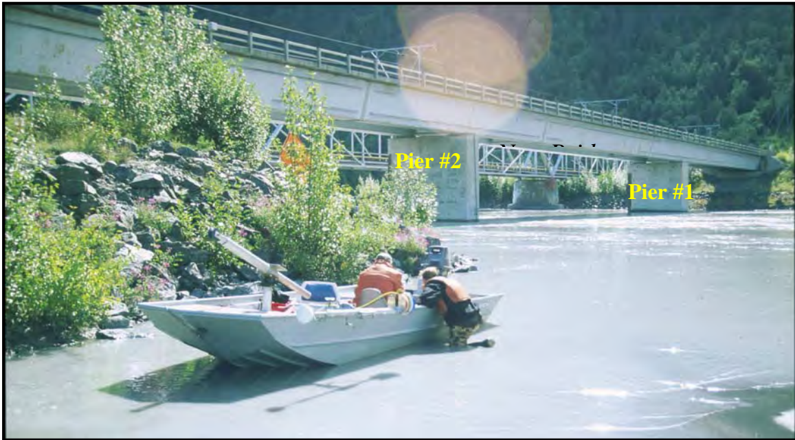
Figure 11. Looking along downstream face of the new Old Glen Highway bridge over the Knik River, field crew and survey boat are in shown in the foreground.
