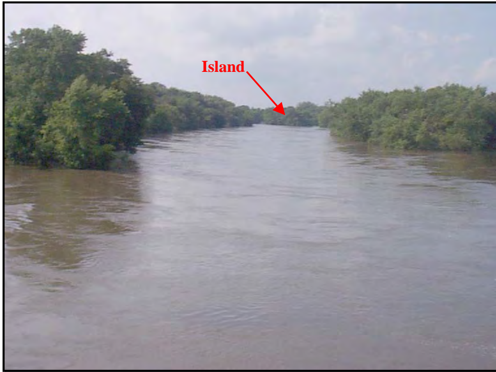
Figure 9. Looking upstream from upstream US 218 bridge over the Cedar River, 7/23/1999.
