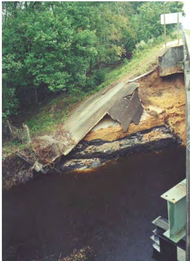
Figure 8. West bound bridge left abutment.
