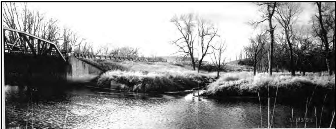
Figure 9. Looking at upstream right abutment and embankment of U.S. 12 bridge during low-flow prior to April, 1997 flood.
