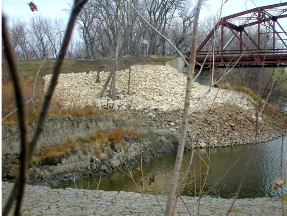
Figure 4. Picture of the re-stabilization done to the left abutment of the S.R 25 bridge over the Minnesota River near Belle Plaine, MN following April, 2001 flood.
