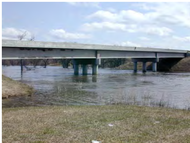
Figure 10. Looking at upstream bridge face from berm on left bank
