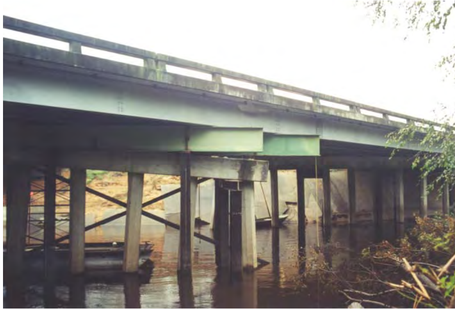
Figure 9. West bound left pile group with temporary steel soldier piles.
