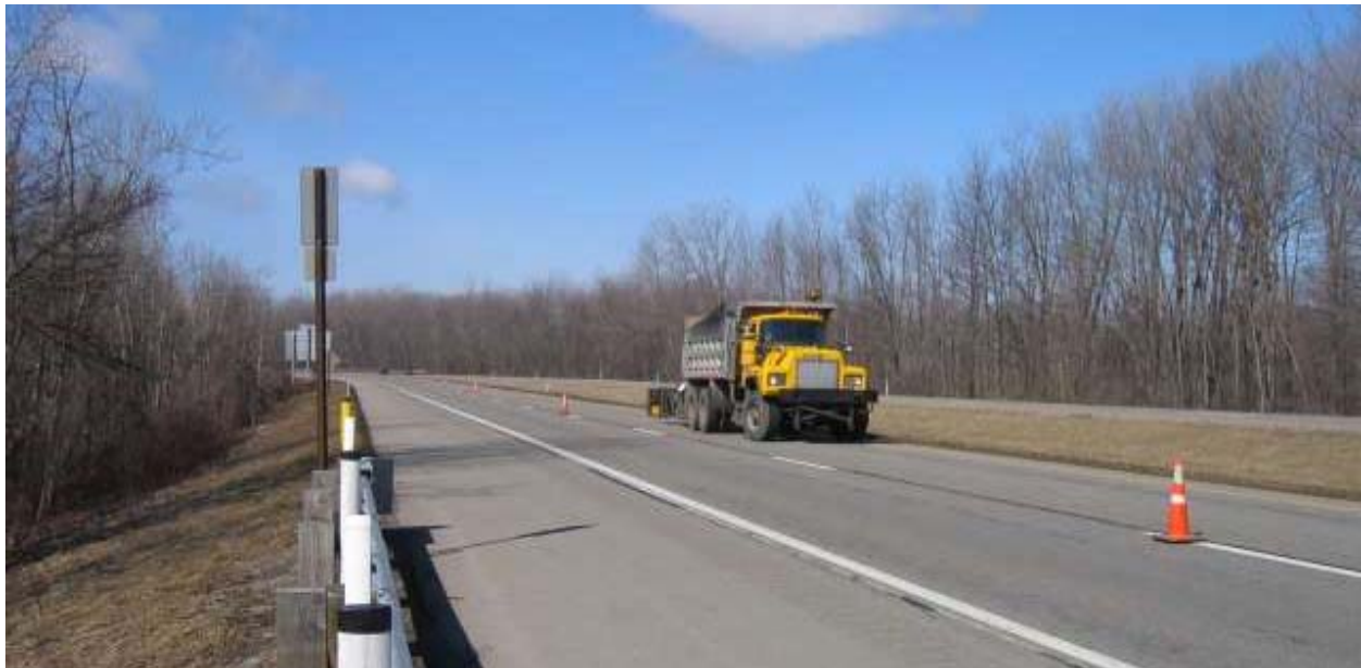
Figure 3. Crash Truck Protecting Operators in a Lane Closure.
