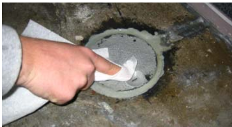
Figure 9. Cleaning Pavement Sensor Depression with a Paper Towel.
