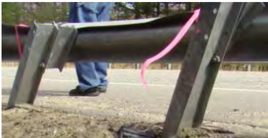
Field Example of Rail Crush
