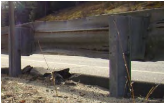
Field Example of Rail Flattening
