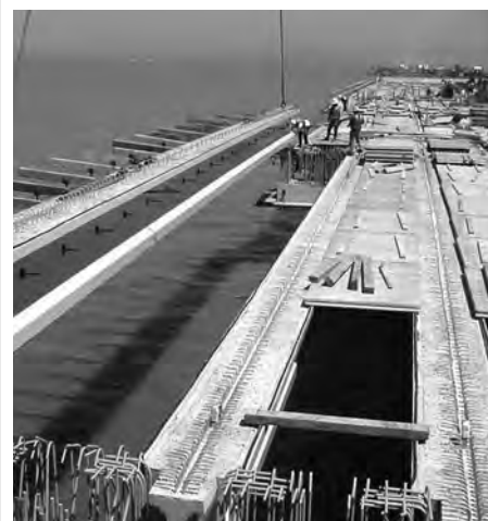
NCHRP research helps California advance accelerated techniques in seismic areas. (Image courtesy of Caltrans)
