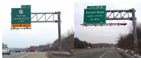
Design differences between traditional (left) and LRFD-based support designs are immediately apparent.
