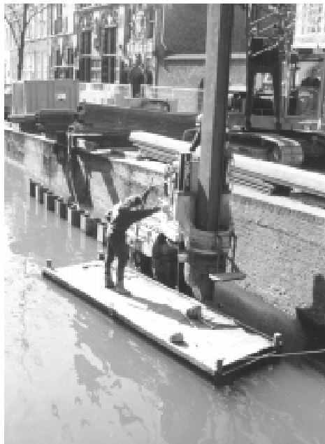
Sheetpiles being installed for canal wall maintenance in Delft, the Netherlands.
