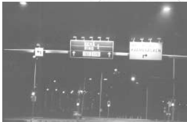
Figure 3. Microprismatic sheeting material on overhead signs in Finland.
