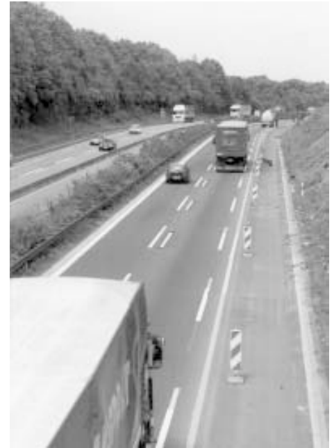
Figure 1. Both lanes have been narrowed in advance of a work zone in Germany, and trucks are restricted to the somewhat wider right lane.
