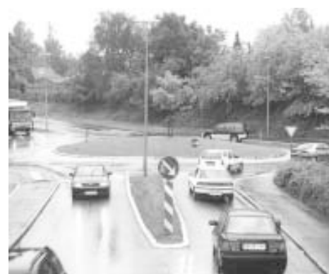
Figure 4. Medium-size roundabout in Denmark.
