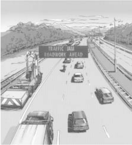
Figure 2. Germany uses yellow markings to delineate travel lanes in work zones; the white markings are left in place, and motorists are taught that yellow markings take precedence over white markings.
