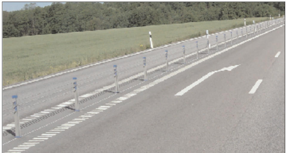
This 2+1 roadway in Sweden features an alternating passing lane with a cable barrier to encourage drivers to pass safely.
