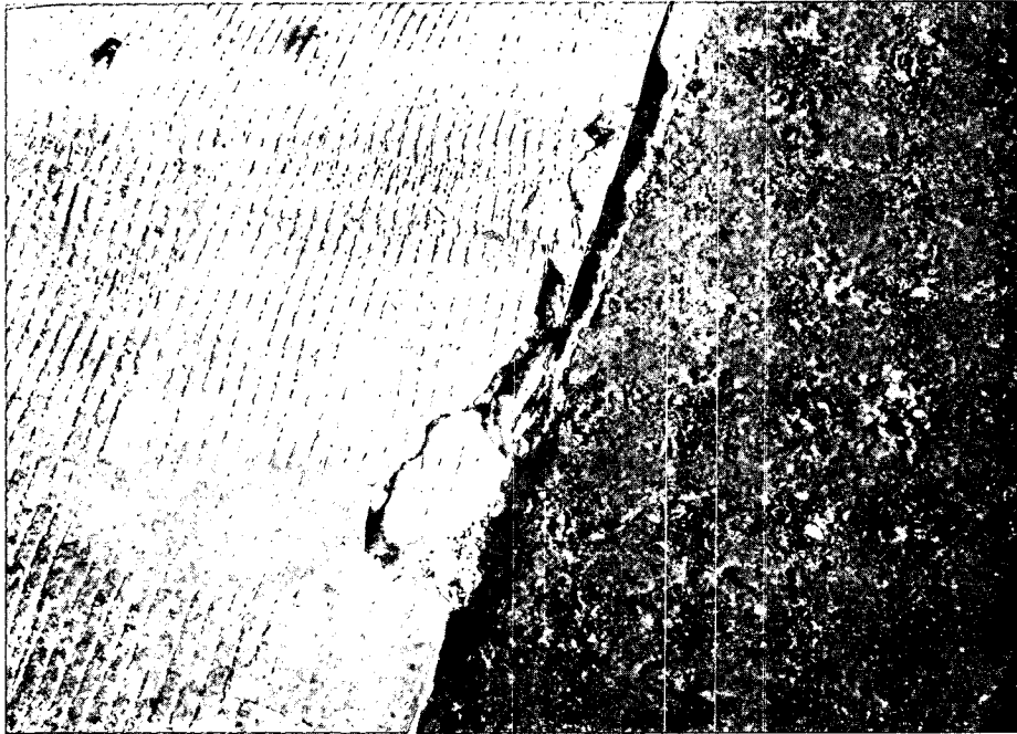
Figure A.13. Cracking at south joint of SFC overlay on I-270 at Site no. 2.
