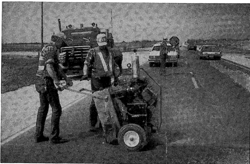
Figure 17. Random crack saw with 8-in (203-mm) diamond blade
