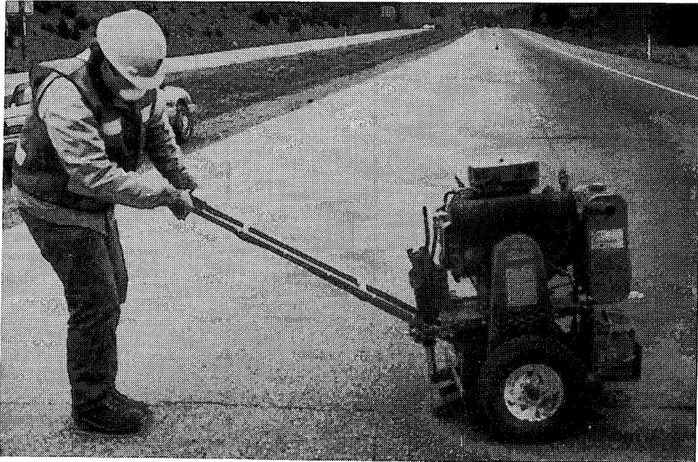
Figure 16. Carbide-tipped rotary-impact router
