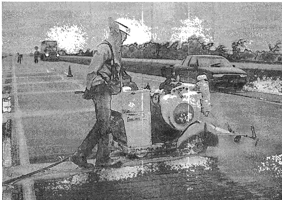
Figure 10. Joint-sawing operation
