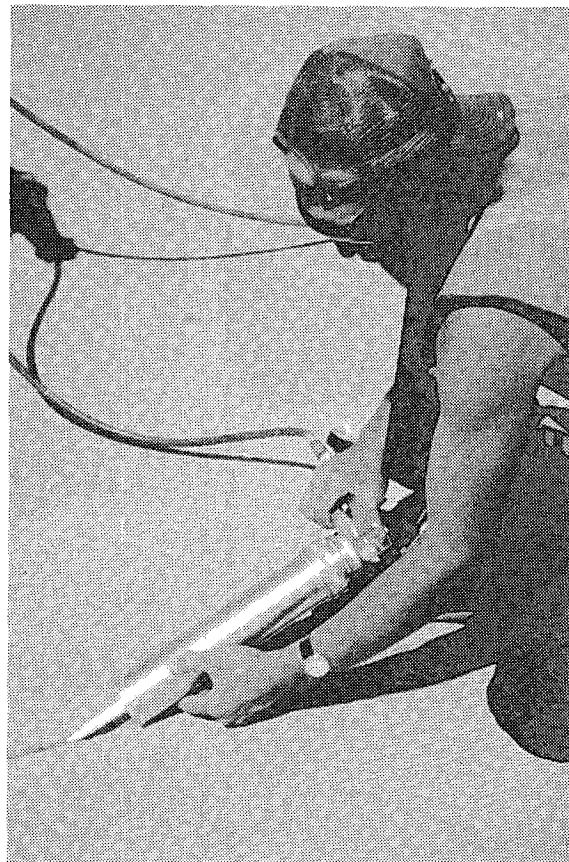
Figure 20. Silicone sealant installation
