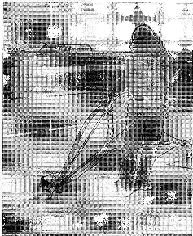
Figure 13. Sandblasting operation
