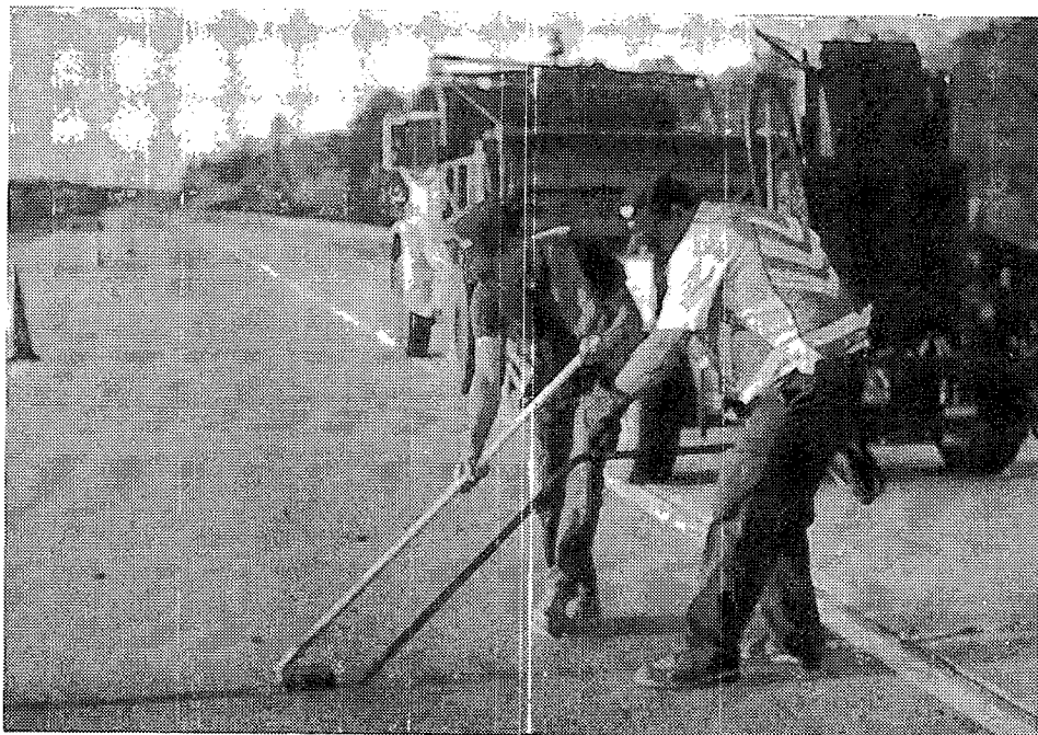
Figure 18. Overbanded sealant installation
