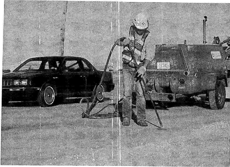
Figure 14. Airblasting operation
