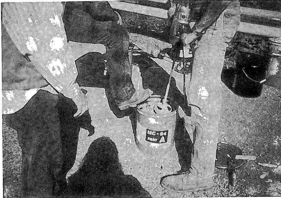
Figure 11. Mixing of MC-64
