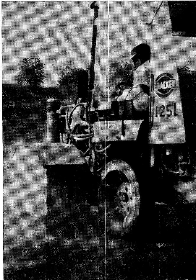
Figure 7. Carbide-tipped, cold-milling machine
