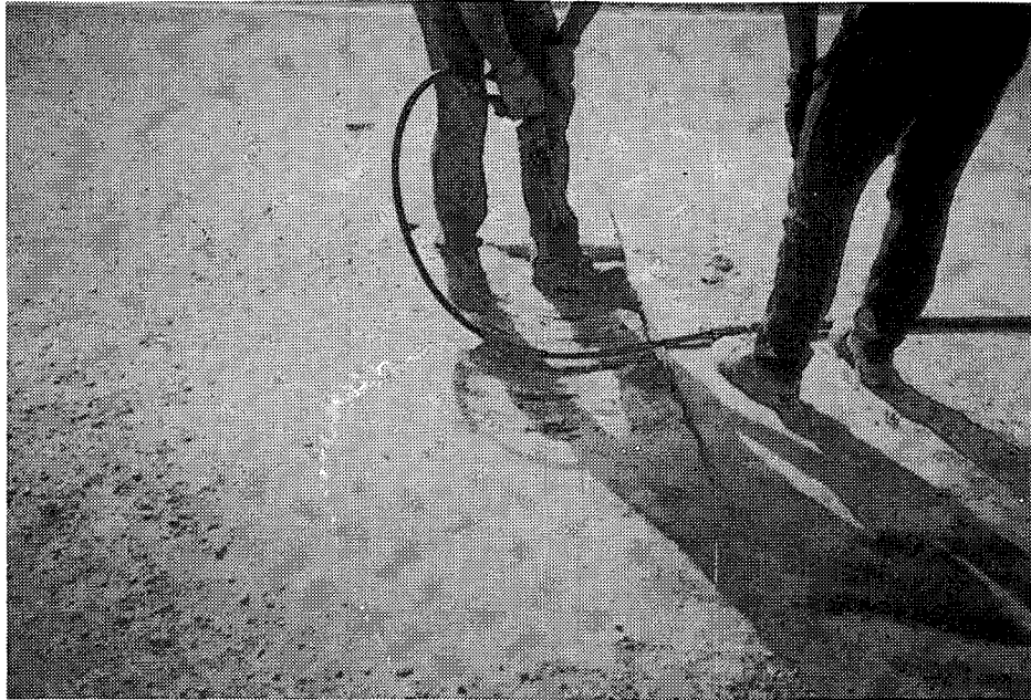
Figure 8. Corners of patch being removed after milling
