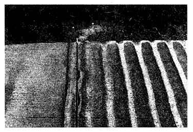
• When the joint has a spall or a saw cut that leaves an enlarged area, an extra backer rod or larger backer rod should be installed before applying sealant. If self-leveling sealant is used, a stiffer version of the same material should be placed over the backer rod with a caulking gun applicator to provide a seal over the backer rod. Otherwise the self-leveling material will flow around the backer rod and develop an improper joint seal.
