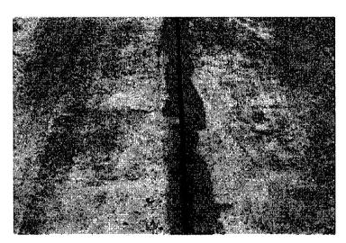
• Applying the sealant to the proper depth in the saw cut will yield a smooth, clean joint to prevent infiltration of surface water and intrusion of incompressible sand and rock particles.
