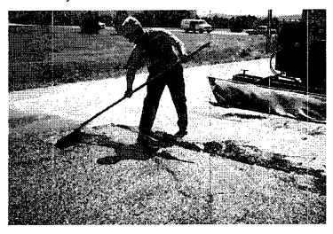
•Roads with superelevated curves make it difficult to control the slurry spreader box to provide for good flow of the slurry mix. Because the mix has a very fluid character, the mix tends to flow to the low side of the box rather than to be evenly distributed along the box. Slurry mix tends to flow out from under the low end of the box. When the low end is on the inside of the roadway curve, the slurry mix tends to flow out onto the shoulder. Keeping the edge of
