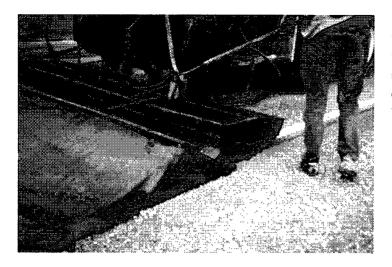
the spreader box on the edge of the paved lane will limit the spreading of the slurry mix onto the shoulder on super- elevated curves. Newer equipment with augers in the spreader box can minimize this problem.
