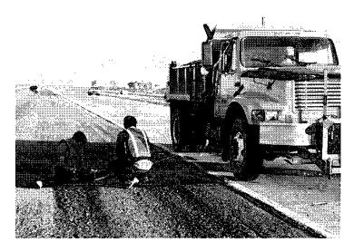
• The contractor should use a deflection measuring device while the grout is being pumped under the slab to ensure that the slab is not lifted by the grout.
