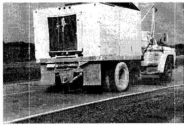
• During grout injecting, the flow of grout out of adjacent holes must be monitored. Injecting too much grout into the void can lead to pumping grout into edge drain systems or lifting of a slab, which will create new voids adjacent to those filled and lead to cracked slabs.
