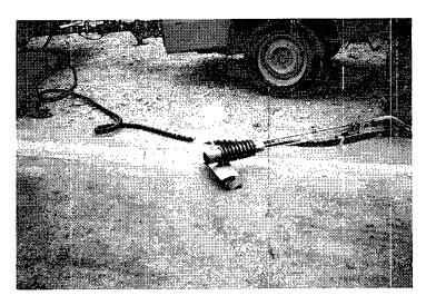
broom the surface with a power broom, blow debris out of the cracks with only compressed air, and then use the hot-air lance to prepare the crack for the sealant.
