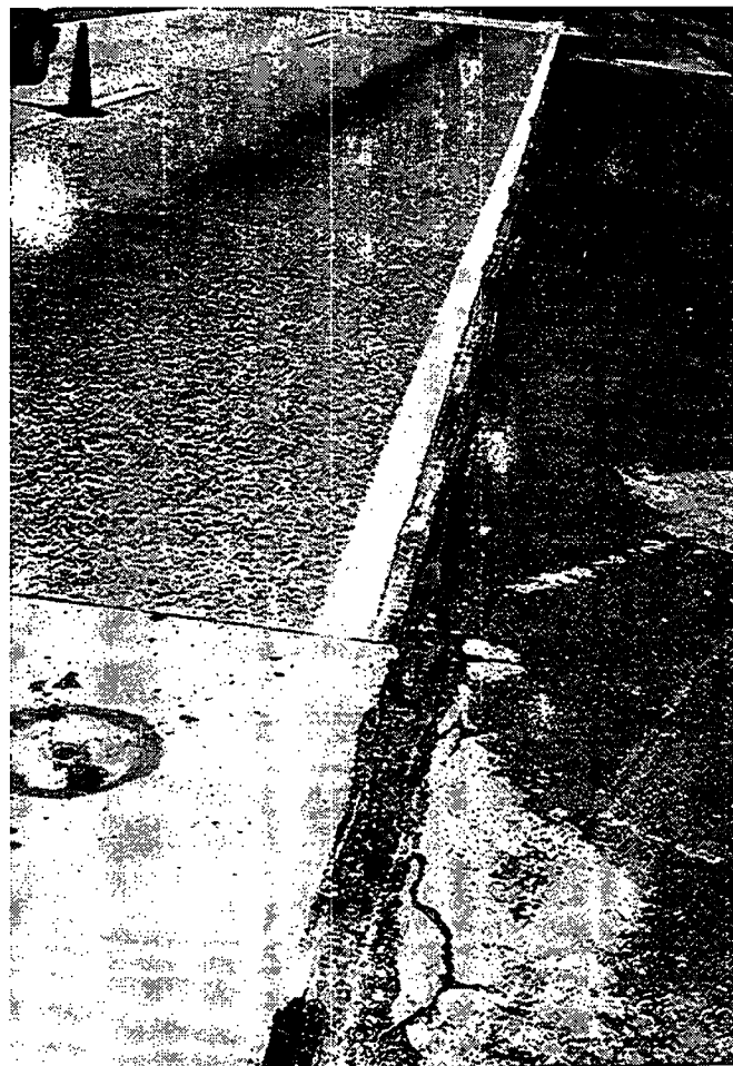
(b) Problems with concrete-asphalt joint
