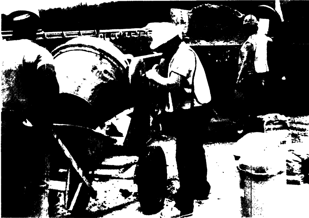
a. Cement, sand, coarse aggregate, and water are batched at site
