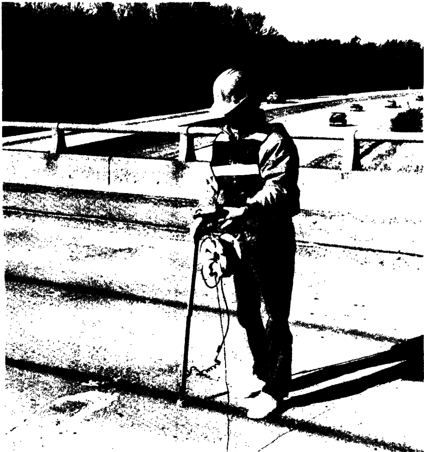
Figure 2. Measuring Static Half-Cell Potentials of Embedded Steel
