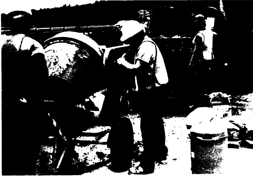
a. Cement, sand, coarse aggregate and water are batched at the site
