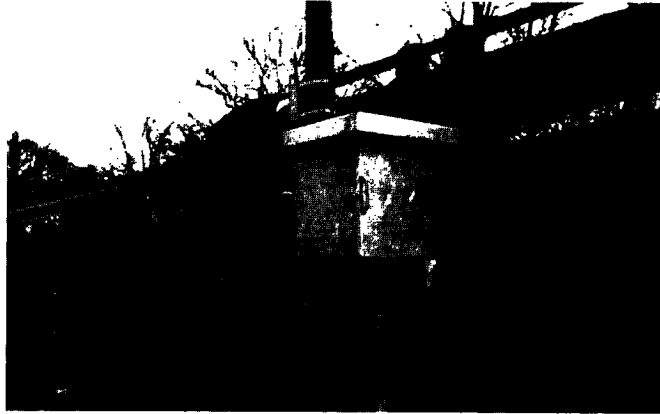
Figure 75. Pole-mounted, air-cooled rectifier installed adjacent to the bridge.
