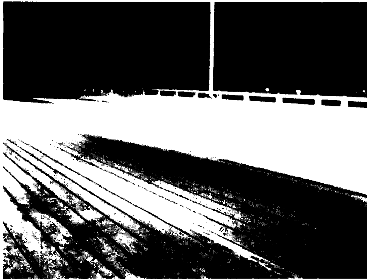
Figure 36. Slots ready for anode installation.
