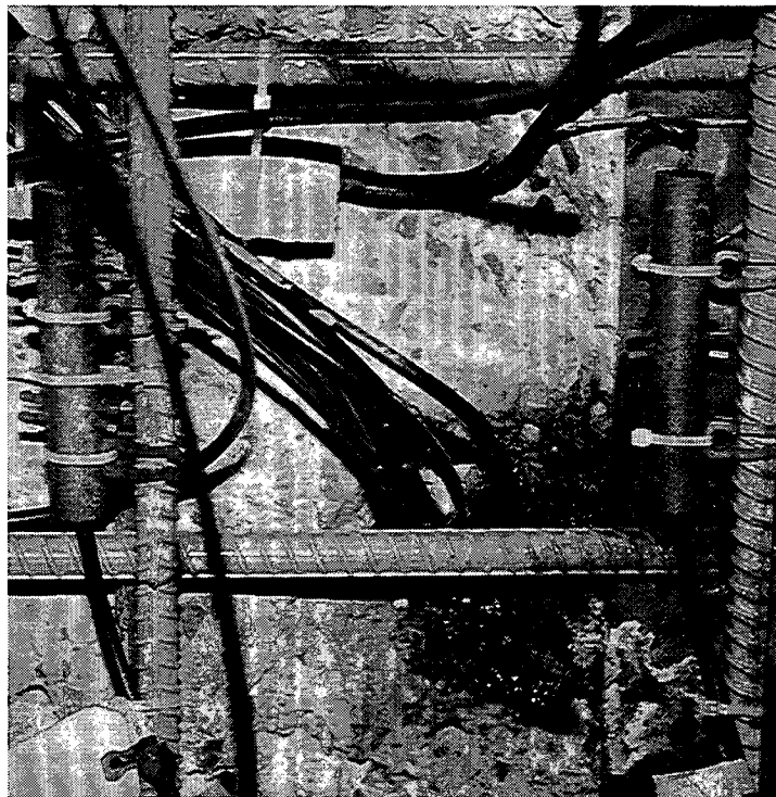
Graphite Half Cell and Rebar Probe in Place
