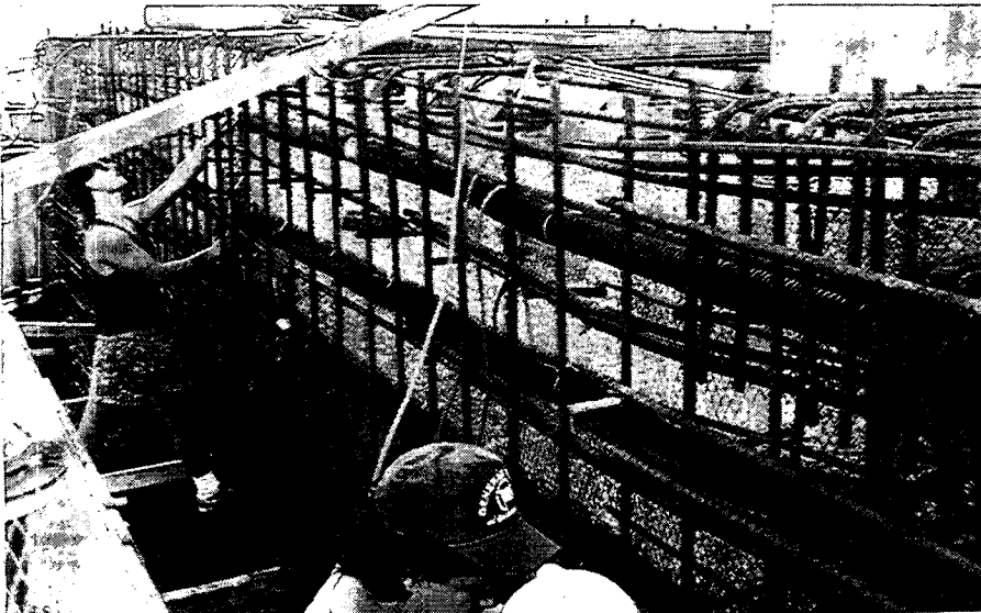
Post-tensioning Duct and New Steel in Place
