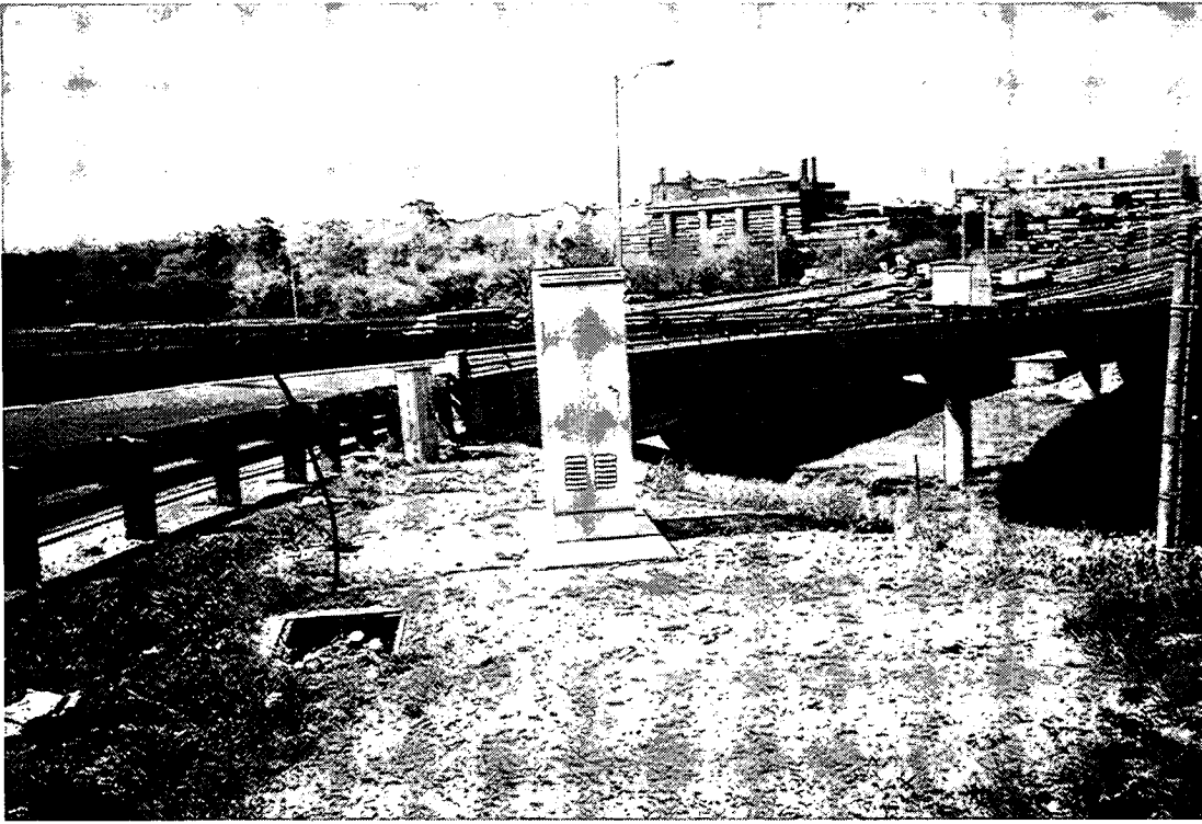
Overall View of the Structure
