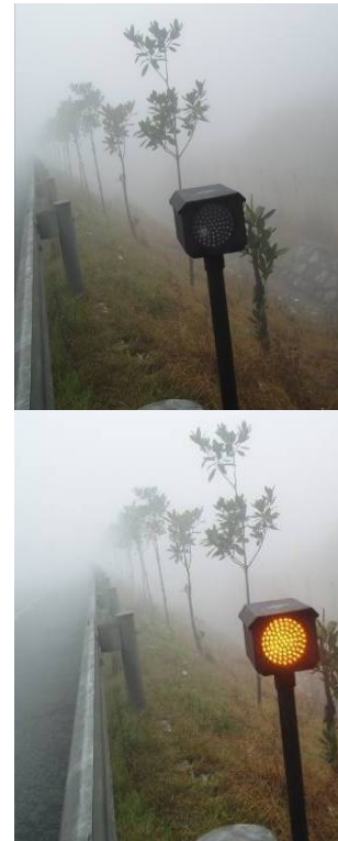
Fog Lamp and Structure
