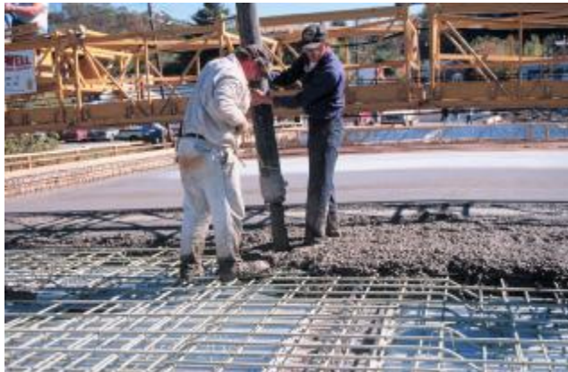
Figure 38. Using self-consolidating concrete
