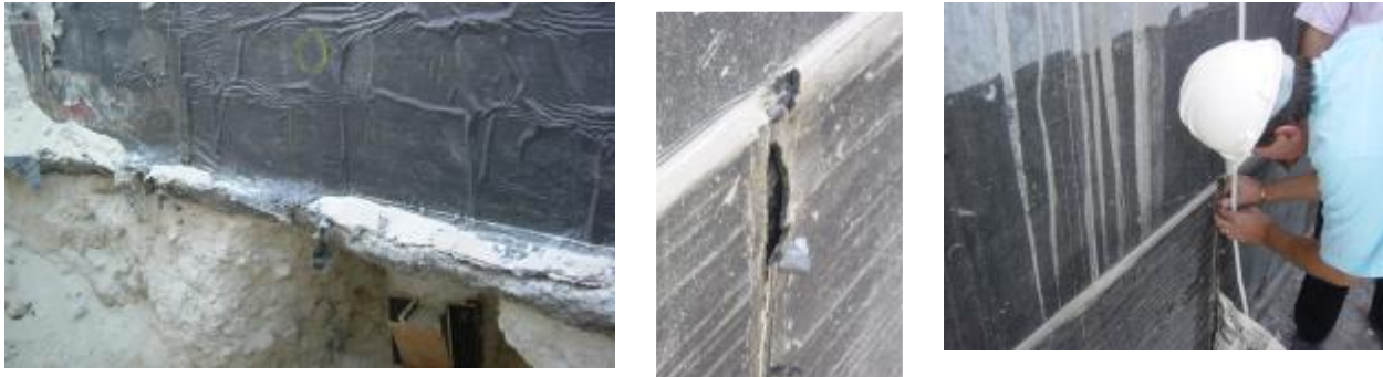
Figure 78. A concrete surface covered by an asphalt membrane
