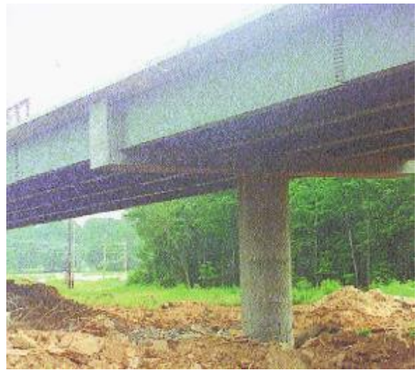
Figure 65. Typical post-tensioned concrete integral bent cap with a single column pier (Wasserman 1997) (courtesy of Tennessee DOT and NSBA).
