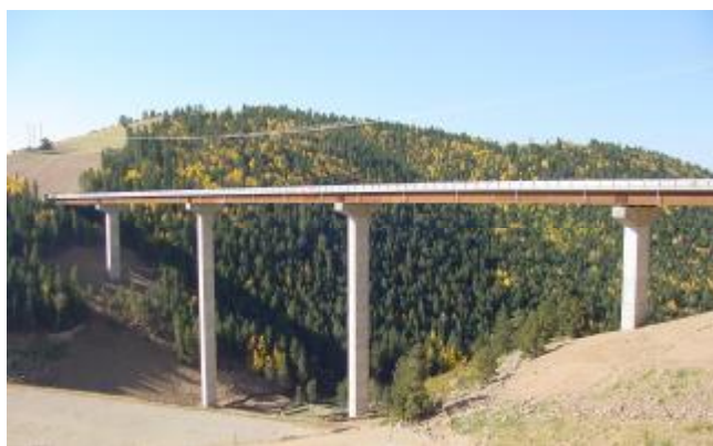
Figure 55. A long continuous steel bridge with joints only at the abutments
