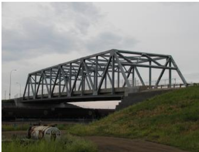
Figure 19. “Metalized” truss bridge over rail yard in South Dakota to minimize maintenance
