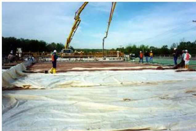
Figure 39. Curing concrete deck
