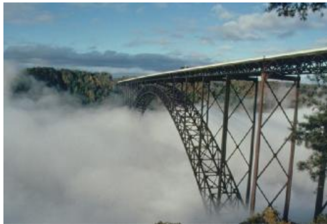
Figure 20. The New River Gorge Bridge (above) in West Virginia is constructed of Weathering Steel
