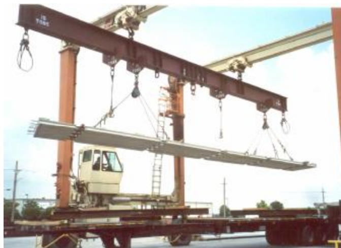
Figure 32. Deck panel being placed for transport
