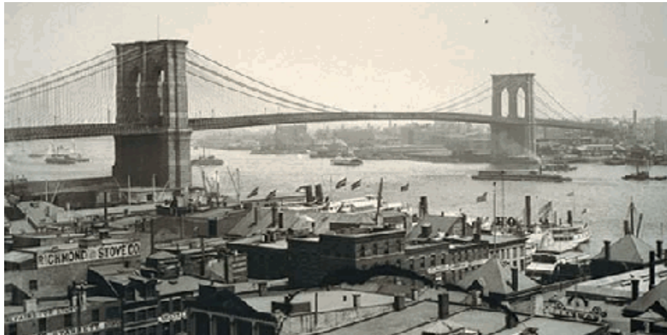
Figure 10. The Brooklyn Bridge from the South Street Seaport, circa 1890
