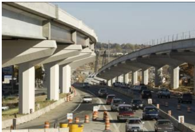
Figure 24. Multi-span precast I girder bridge, made continuous for Live Load.
