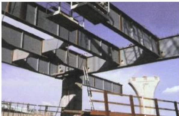
Figure 66. Straddle bents with integral steel pier caps (Abu-Hawash et al. 2005) (courtesy of Iowa DOT, HDR Engineering and NSBA)
