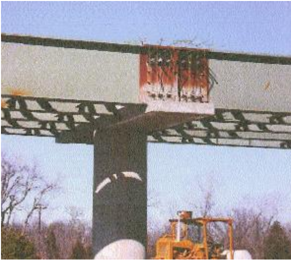
Figure 65. Typical post-tensioned concrete integral bent cap with a single column pier (Wasserman 1997) (courtesy of Tennessee DOT and NSBA).
