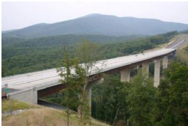
Figure 21. These steel girders are fabricated from Weathering Steel
