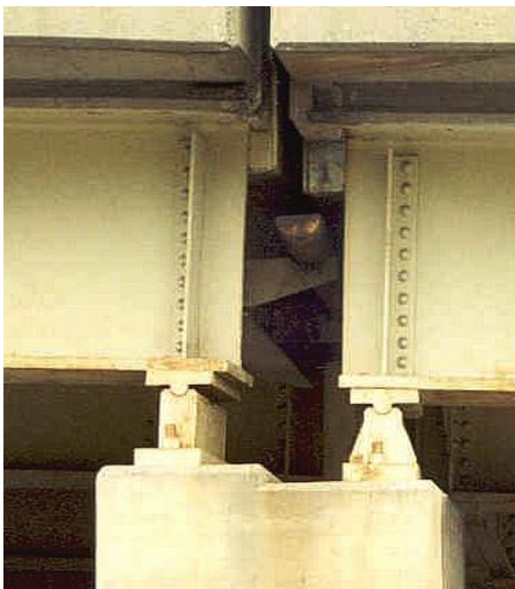
Figure 59. Fabricated steel bearing with rockers
