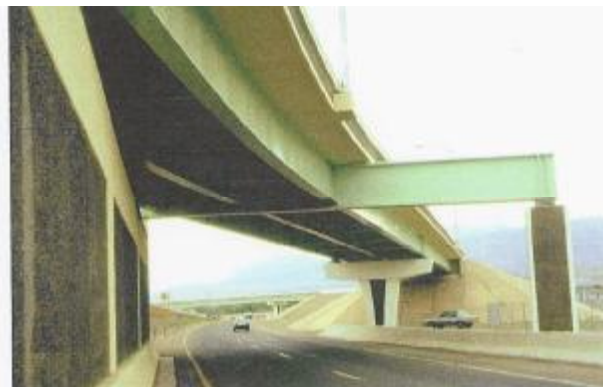
Figure 66. Straddle bents with integral steel pier caps (Abu-Hawash et al. 2005) (courtesy of Iowa DOT, HDR Engineering and NSBA)
