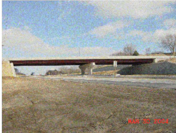
Figure 33. Completed Skyline Bridge
