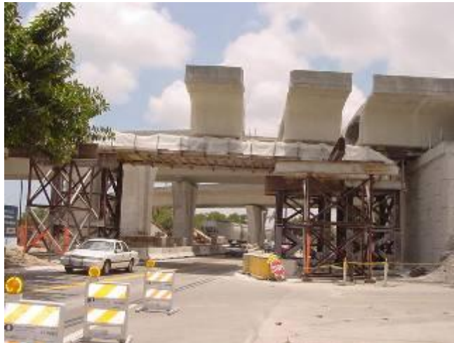
Figure 13. De-construction of Segmental Bridge, in Florida, due to Functional Obsolescence
