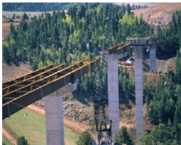
Figure 17. Typical I-girder steel bridge
