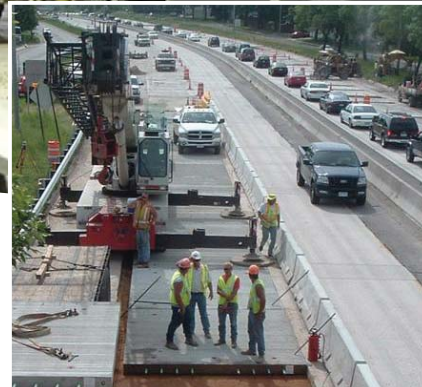
Left: Prestressed PCP, Virginia DOT; Right: Jointed PCP, Minnesota DOT.
