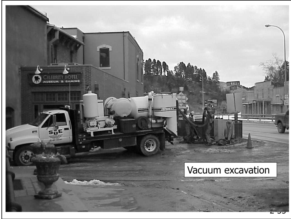
This picture shows the vacuum excavation to expose the utilities.
