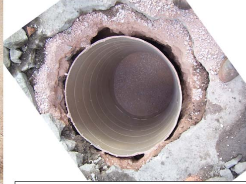
Redesign using 30" sonotube (longer, narrower footing)
