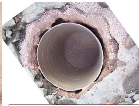
Redesign using 30" sonotube (longer, narrower footing)
