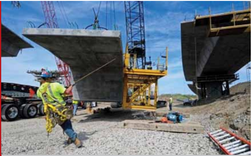
Wrangling a precast section on Highway 62 in Minneapolis. Photo by David Gonzalez, Minnesota DOT
