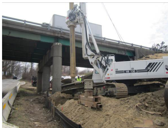
Figure 5. Drilled Shaft Soil Auger.
