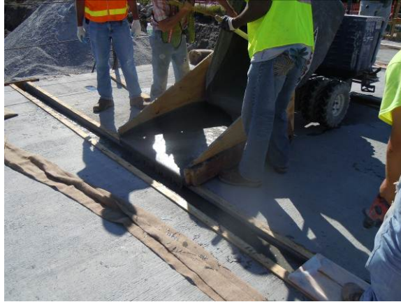
Figure 11. Placing of UHPC.
