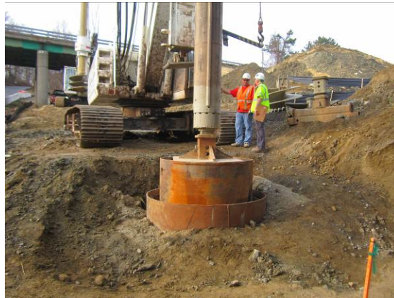
Figure 6. Drilled Shaft Core Barrel.
