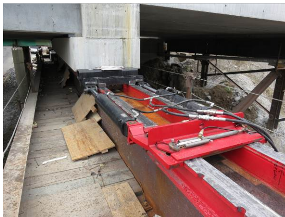
Figure 15. Hydraulic jacks and gripper assembly.
