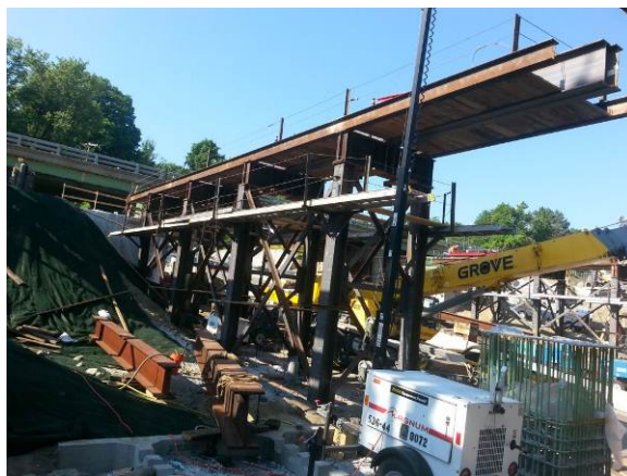
Figure 9. Primary bent. Source: NYSDOT.
