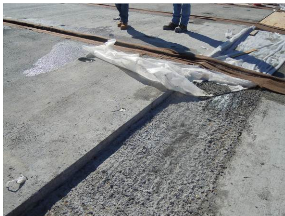
Figure 19. Step resulting from NEXT beam camber.
