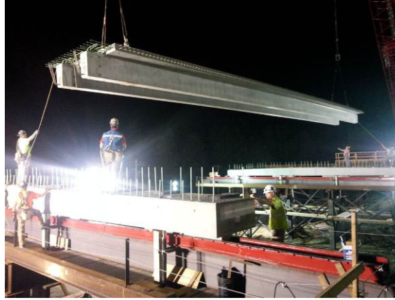
Figure 10. Setting of first NEXT beam. Source: NYSDOT.
