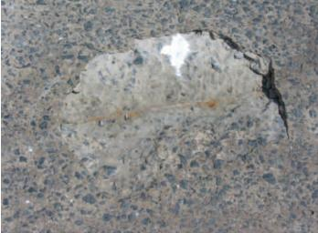
Figure 2.1. Deck deterioration.
