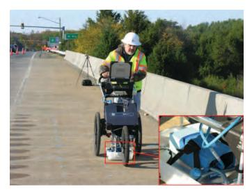
Figure 3.10. GPR testing.
