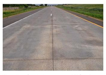
Figure V.20. Streaked appearance of EAC surface caused by caking of paste by brush machine wheels.
