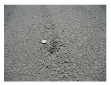
Figure V.19. Area of EAC surface that was not closed before brushing.
