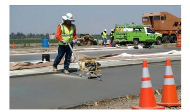
Figure G.32. Early entry saw cutting joints on Lane D.
