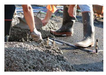
Figure G.28. Hand packing concrete around instrumentation.
