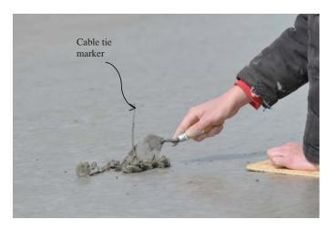
Figure H.3. Cable ties attached to the dowel so that the sensor locations could be easily located.
