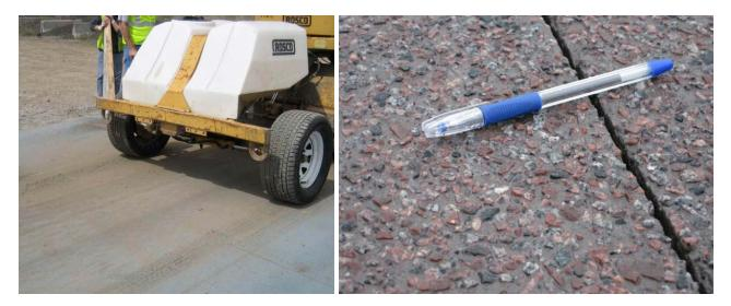
Figure F.35. Surface after first pass with brush (left); finished EAC surface after wash (right).
