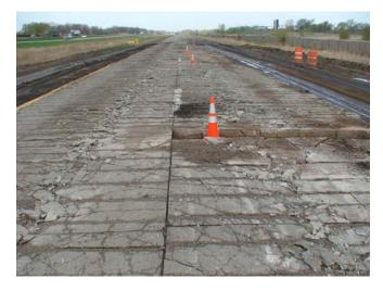
Figure F.5. Existing concrete pavement following breaking using the guillotine crusher.
