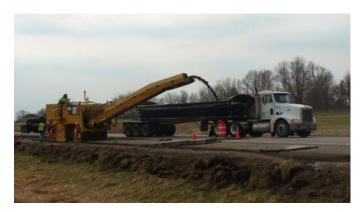
Figure F.8. Milling of existing HMA shoulder to be used as recycled asphalt pavement (RAP) in the construction of new HMA shoulders.
