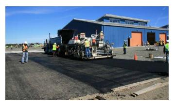
Figure G.45. Paving top lift 2-in. (50-mm) RHMA-G in Lane D, Section 1.
