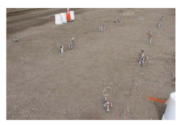
Figure H.23. Photograph of the sensors installed in Slabs 1 and 2 before paving.
