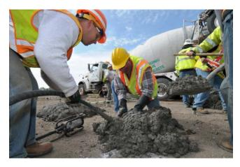
Figure H.26. Concrete was placed around the sensors to protect the sensor before the passing of the paver.
