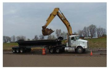
*Figure F.7. Transportation of existing concrete pavement for recycling.*
