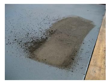
Figure V.16. Evaluating brushing readiness of the EAC surface with a push broom.
