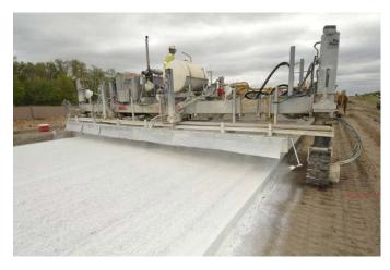
Figure F.23. Applying curing compound to the surface of the PCC to control surface drying of the PCC and minimize early-age distresses.
