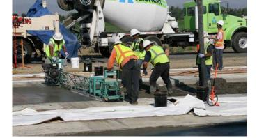
Figure G.33. Burlene in place on Lanes A and C, while Lane B is paved on Day 2 (Burlene has been temporarily pulled back to allow screed to pass).
