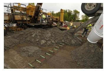
Figure F.32. Placement of the lower PCC mix.
