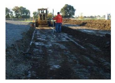
Figure G.5. Initial excavation of test track subgrade.
