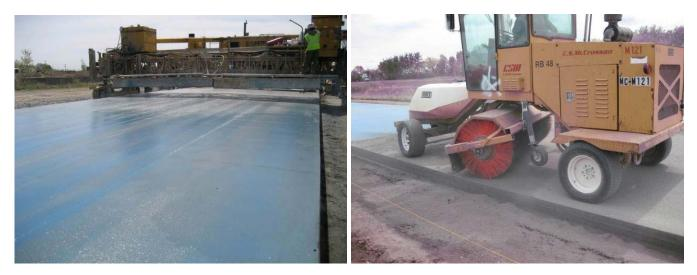
Figure F.34. Treated surface and finishing platform (left); equipment for EAC brushing (right).
