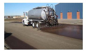
Figure G.12. Further pass of prime coat application truck.
