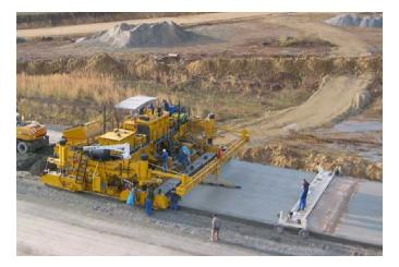
Figure B.5. Two-lift slipform paving in the Czech Republic.
