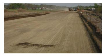
Figure F.13. Trimmed and compacted subgrade.
