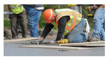
Figure H.13. Installation of the static strain gauge for the upper concrete layer for Cells 71 and 72.
