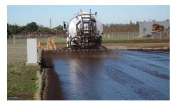
Figure G.13. Completed application of prime coat.
