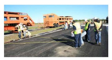
Figure G.43. Measurement of the positions of CTL strain gauges on first lift of PG 64-28PM, before placement of second lift.
