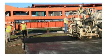
Figure G.38. Start of PG 64-28PM placement following application of tack coat.
