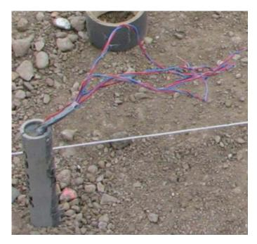
Figure H.4. Thermocouples installed in Cell 70.
