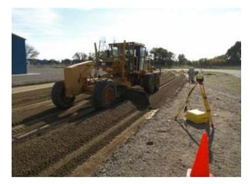
Figure G.9. Aggregate base grading.
