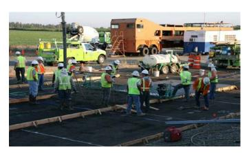
Figure G.29. Motorized screed on Lane C, Day 1 of PCC paving.
