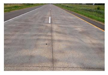
Figure V.21. Marbled EAC surface resulting from saturation during construction.
