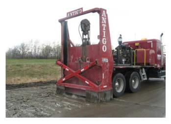
Figure F.4. Guillotine crusher breaking existing concrete for recycling into the PCC layer of the HMA/PCC composite pavement.
