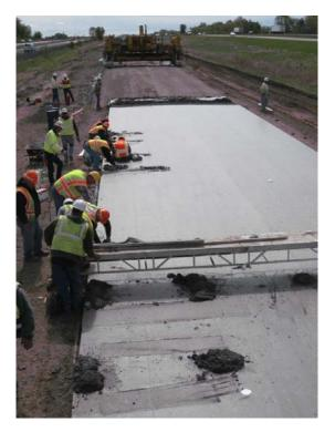
Figure H.29. Installation of sensors for the upper PCC layer after passage of the first paver. Photograph taken from the second paver.
