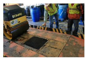
Figure G.51. Compaction of ingots with rolling wheel compactor.
