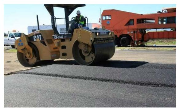
Figure G.46. Compaction of 2.0-in. (50-mm) second lift RHMA-G on Lane C.
