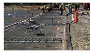
Figure G.24. Track overview showing sensor wires fixed to track.
