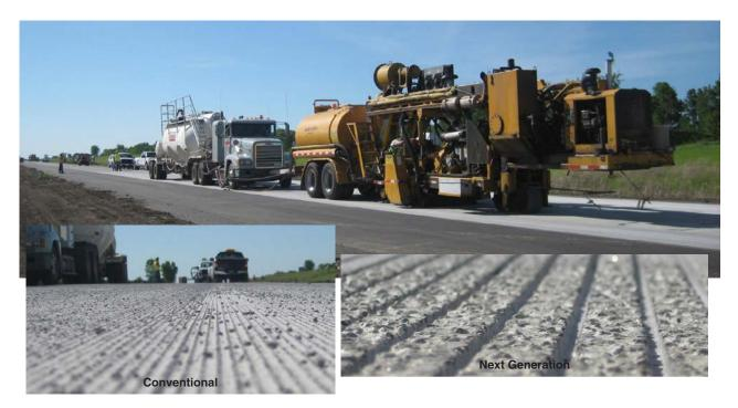
Figure F.37. The initial learning portion of the EAC texture was diamond ground using conventional grinding in the passing lane and next-generation grinding in the driving lane.
