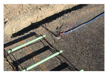
Figure G.23. Cable-fastening process showing a combination of Bituthene and nail methods.
