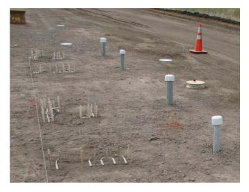
Figure H.16. Example of the vertical PVC pipe where the dynamic strain gauges were stored until after the pass of the first paver for Cells 71 and 72.
