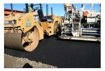
Figure G.40. Compaction and placement of RHMA-G in Lanes C and D.
