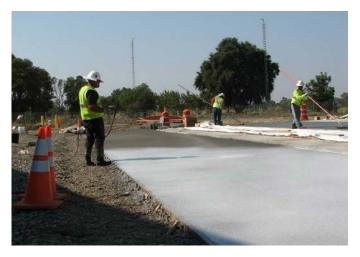
Figure G.31. Applying the first coat of curing compound on Lane D.
