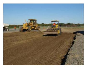
Figure G.7. Placement and compaction of test track subgrade.
