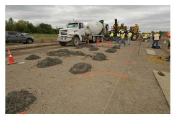
Figure H.27. Mounds of concrete placed around the sensors before the passing of the paver.
