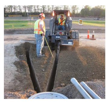
*Figure F.14. Installing conduits to carry and protect the instrumentation cables.*
