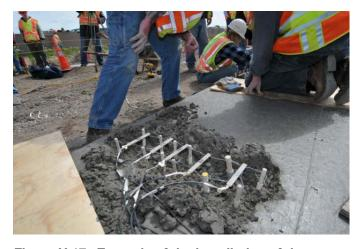
Figure H.17. Example of the installation of the dynamic strain gauges in the upper concrete layer for Cells 71 and 72.
