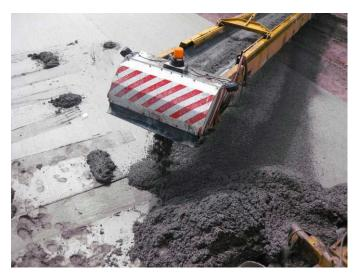
Figure F.33. Placement of the upper PCC mix on the lower PCC layer.
