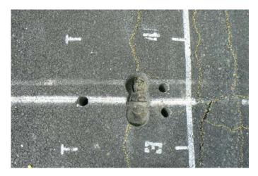
Figure K.57. Top view of Section 614HB taken near Joint J1 showing slab cracking underneath.
