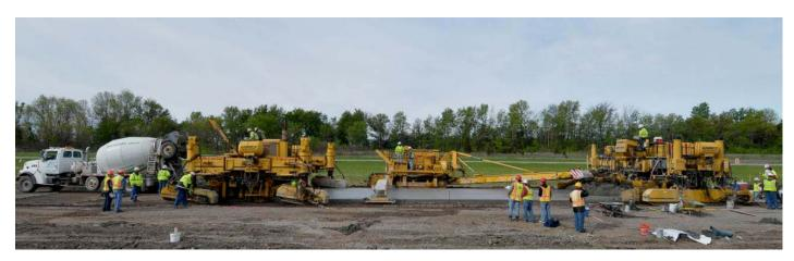
Figure F.25. Paving train constructing R21 test sections along I-94 at MnROAD. Pictured from left to right are the mixer truck, first paver, belt placer, and second paver.
