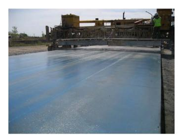
Figure V.15. Streaked application of MBT Reveal on the demonstration slab.
