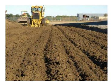
Figure G.6. Scarification and drying of test track subgrade before grading and compaction.
