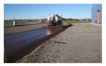
Figure G.11. Initial pass of prime coat application on eastern side of track.
