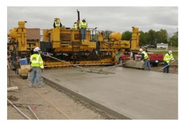
Figure F.21. Finishing the PCC surface to remove surface irregularities.
