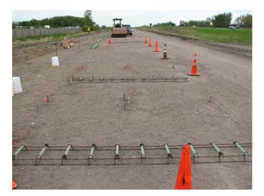
Figure H.25. Photograph of VW, TC, and MC installations in Cell 70 before paving.
