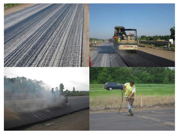
*Figure F.24. Tack coat applied to PCC surface (top left) before HMA paving (top right). Sawing (bottom left) and sealing (bottom right) HMA layer; saw cuts in the HMA were matched to the saw cuts in the PCC below to within 12.5 mm (0.5 in.).*
