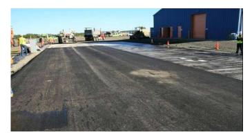
Figure G.39. Completed first lift of PG 64-28PM over Lanes A and B.
