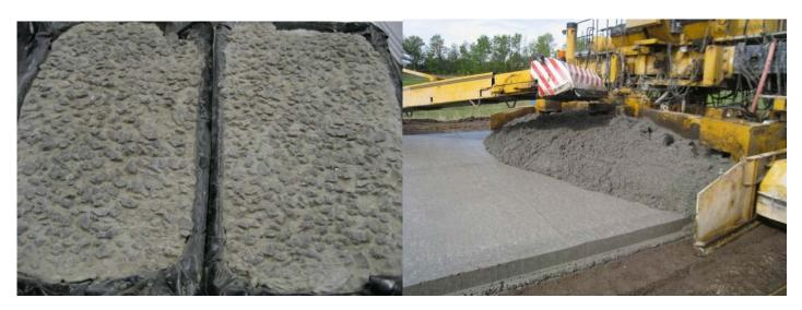
Figure F.29. At left, PCC specimens cast in preparation for the paving and brushing of the PCC/PCC demonstration slab. At right, top surface PCC mix being placed in front of the second paver on site at MnROAD.
