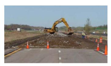
Figure F.6. Removal of existing concrete pavement for recycling.
