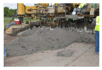
Figure F.20. Placement of PCC layer on the aggregate base.
