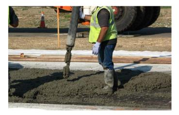
Figure G.27. Pumping concrete on Lane B on Day 2, between completed Lanes A and C.
