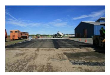
Figure G.41. Completed first lift of PG 64-28PM (left two lanes) and RHMA-G (right two lanes).
