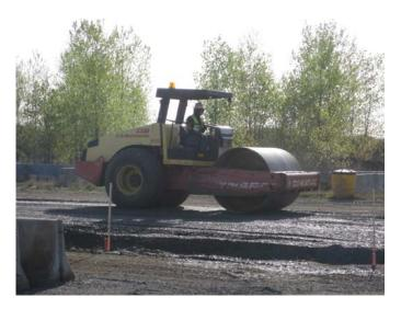
Figure F.12. Compacting the subgrade using a steel drum roller.
