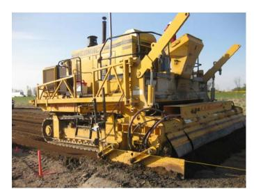
Figure F.11. Trimming the subgrade using a string line and trimmer.
