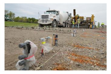
Figure H.28. Photograph of the sensors directly adjacent to the shoulder as the paver approaches.
