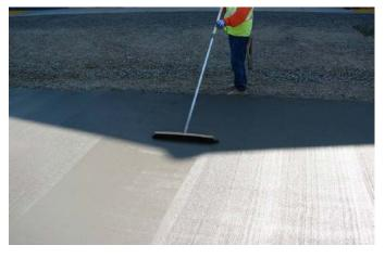
Figure G.30. Texturing the concrete surface.
