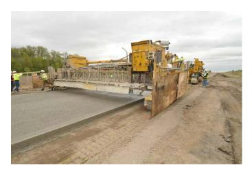
Figure F.22. Tining the PCC surface to provide texture for mechanical bonding between PCC and HMA layers.
