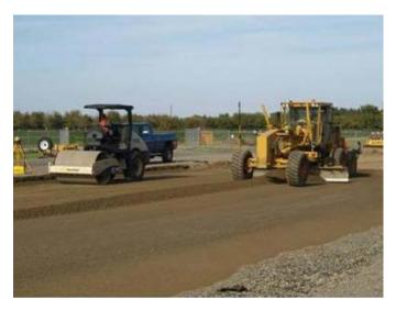
Figure G.10. Compaction and grading of test track aggregate base.
