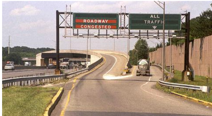
Figure 59. Signage at Entrance Ramps, New Jersey Turnpike (1)
