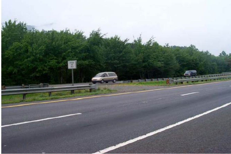
Figure 3. Emergency Crossover on I-40 Near Asheville, North Carolina (1)
