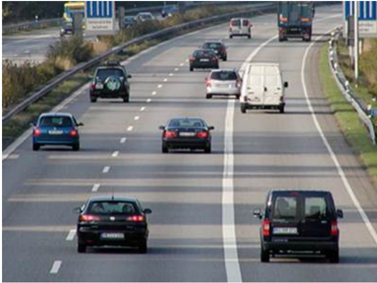
Figure 18. Drivable Shoulder in Germany (1)
