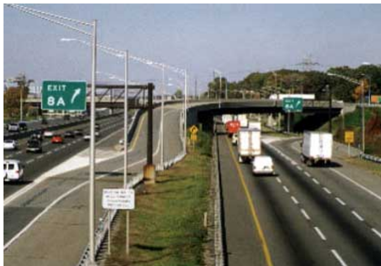
Figure 60. Dual Facilities Along the New Jersey Turnpike (2)
