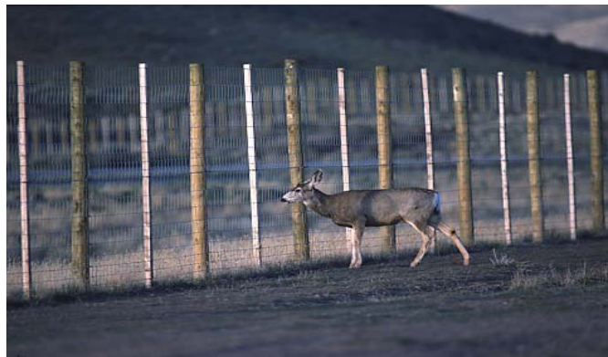
Figure 44. Wildlife Fencing Installed to Keep Wildlife From Crossing Highways (2)
