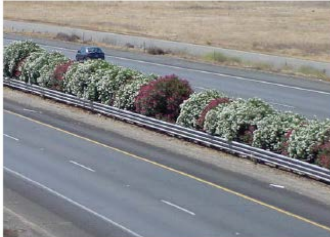
Figure 13. EHMB Created Using Oleander Shrubs (this has been done in California since the 1950s) (3)
