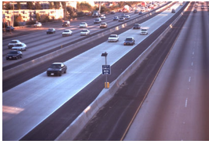
Figure 64. Reversible Lane on I-15 in San Diego, California (3)
