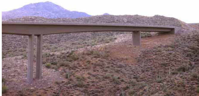
Figure 46. Long Tunnels and Long Bridges Physically Separate Animals From Vehicular Traffic (4)
