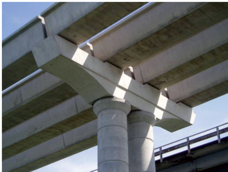
Figure 41. The Use of Precast Materials During Bridge Construction in Texas (2)
