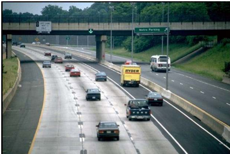
Figure 19. Drivable Shoulder Along I-66 in Virginia (2)
