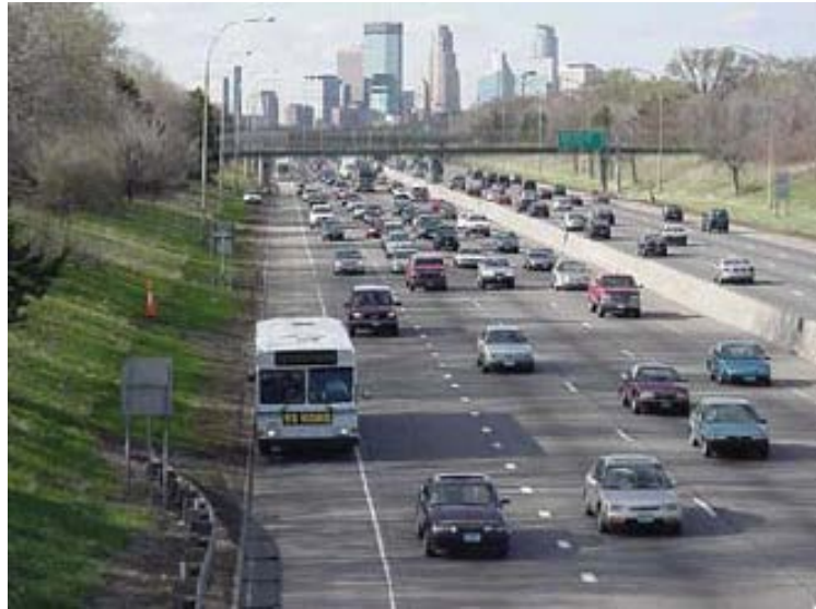
Figure 20. Bus-Only Drivable Shoulder on I-35 in Minneapolis (3)
