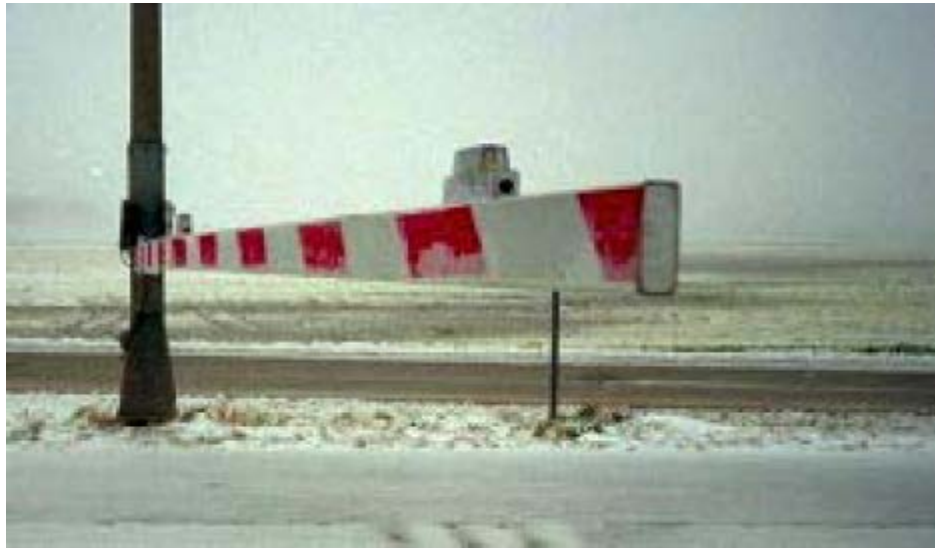
Figure 32. An Automated Gate Used to Close Access in the Event of Severe Weather Conditions (1)
