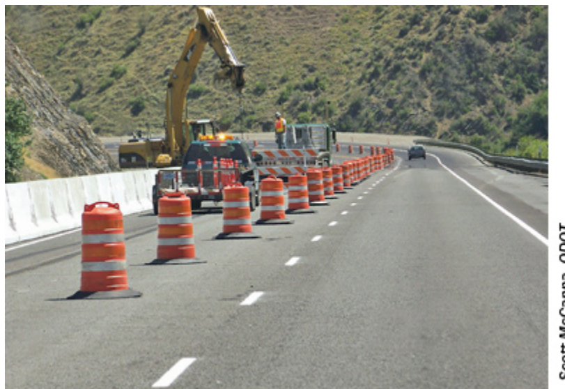
Figure 42. Example of Work Zone Where Access of Slow-Moving Vehicles Will Likely Impede Traffic (1)
