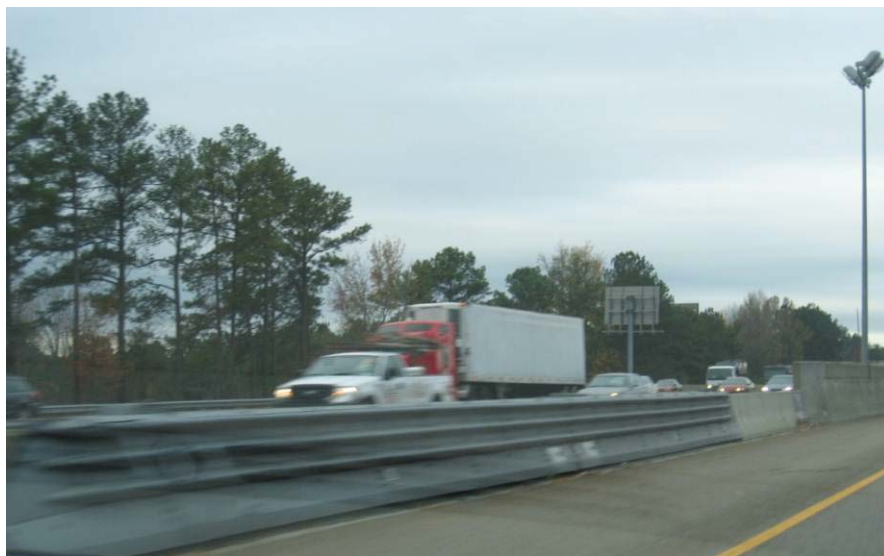
Figure 8. Gated Median Barrier in Atlanta, GA (2)
