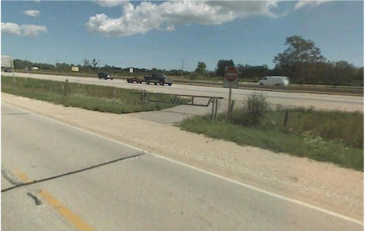
Figure 30. Emergency Access Between Interchanges (I)
