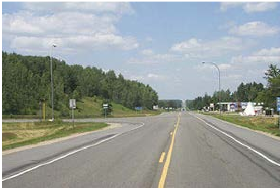
Figure 4. Emergency Crossover in Minnesota (2)
