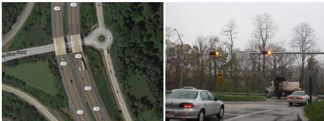
Figure 35. Aerial Image of the Maryland Roundabout (Left), and Photo Showing the Signalized Arterial Leg of the Roundabout (Right) (2)
