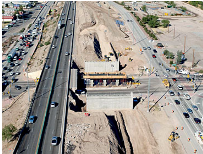
Figure 65. Work Zone Express Lane Along I-10 in Tucson, Arizona (1)
