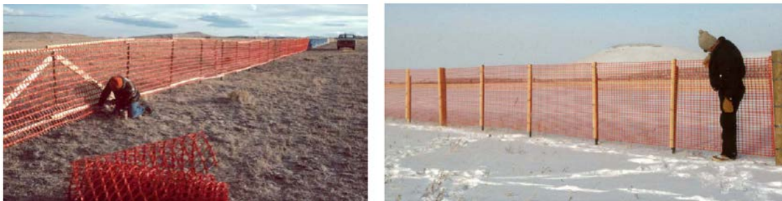
Figure 48. High-Density Polyethylene Snow Fences (I)
