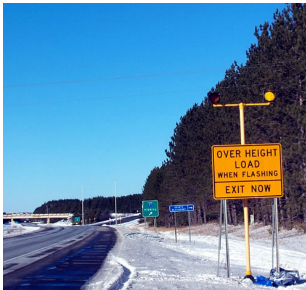
Figure 89. Over-Height Detection System in Minnesota (2)
