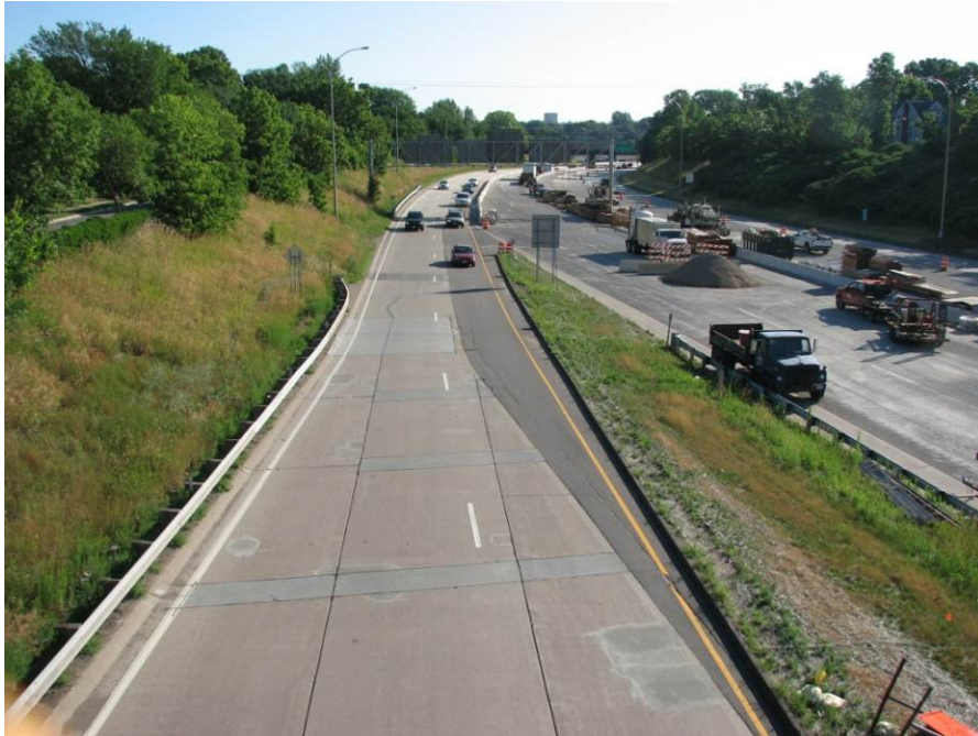
Figure 31. A Two-Lane Off-Ramp in Minnesota (1)
