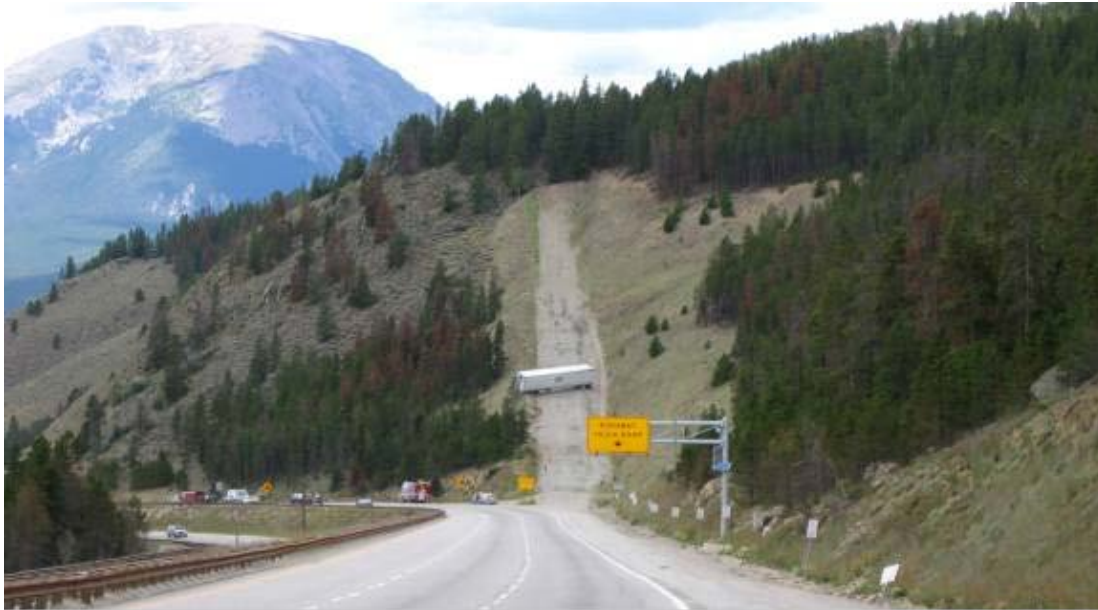
Figure 39. Example of a Gravity Runaway Truck Ramp (2)
