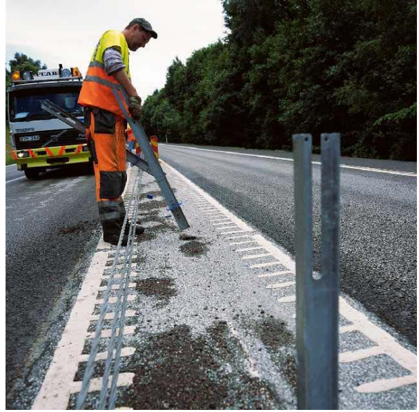
Figure 9. Moveable Cable Median Barrier in Normal State (left) and Collapsed State (right) (1)
