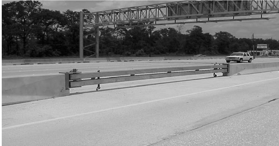
Figure 7. TTI Access Gate (1)
