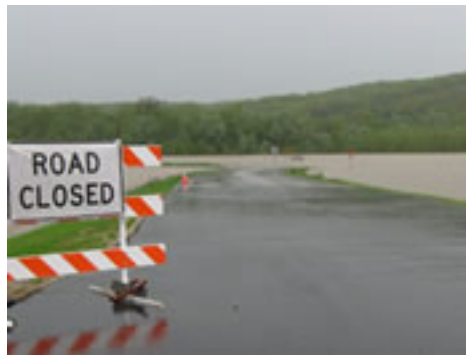
Figure 98. Closed Flooded Roadway (2)
