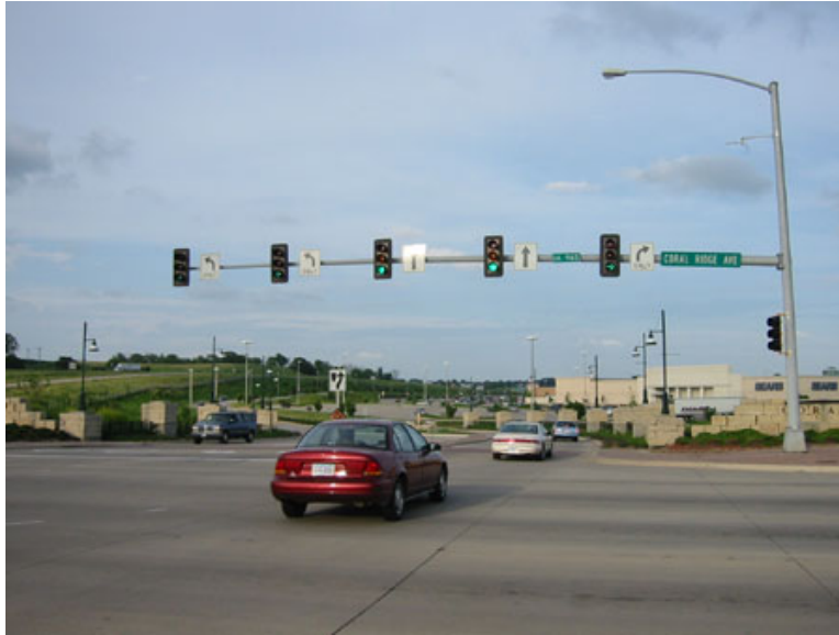
Figure 75. Lane-Aligned Signal Heads (2)
