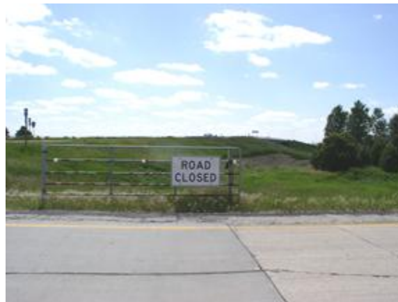
Figure 33. Left-Side Swing Gate on I-35 in Iowa (2)
