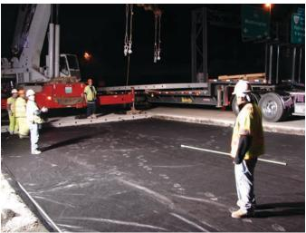
Figure 12.1. Placement of polyethylene sheet or geotextile fabric.
