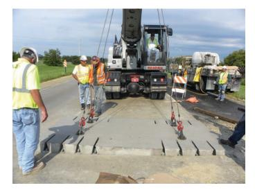
Figure 14.5. Narrow-mouth surface dowel slots.
