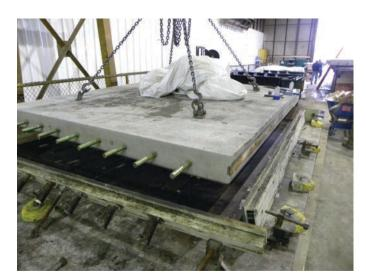
Figure 4.2. Typical four-point lifting of a precast panel.
