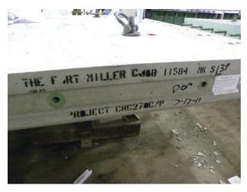
and creep. The dunnage location should be shown on shop drawings. The storage of nonplanar panels may require shimming at the dunnage to accommodate the warp. The upper panels of a stacked tier should not be used as storage areas for smaller panels or equipment.
