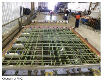
*Figure 9.3. Reinforcement placed in both directions.*
