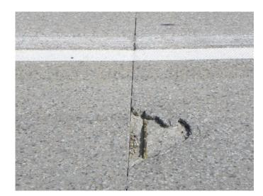
Figure 3.19. Spalling at an intermediate transverse joint on I-57 in Missouri.
