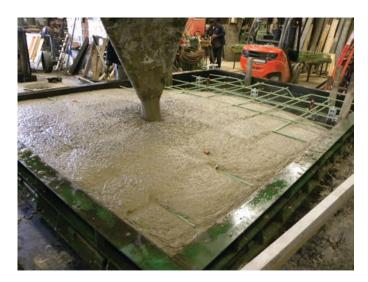
Figure 9.7. Placement processes for slump concrete and SCC.
