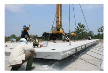
Figure 2.18. Indonesia PPCP installation.
