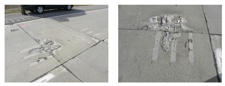
Figure 3.6. Views of a deteriorated panel at the I-675 project (planned for replacement) in Michigan.
