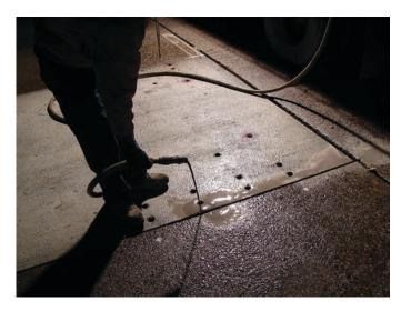
Figure 10.7. Dowel slot grouting.
