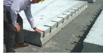
Figure 2.12. Kwik Slab joint interlocking system.
