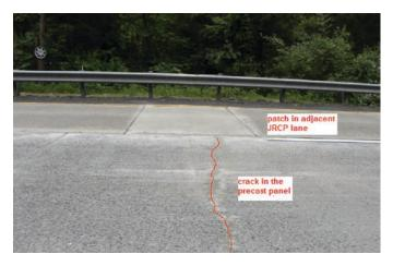
Figure 3.11. Crack in a precast panel associated with a patch in the adjacent lane on I-66 in Virginia.
