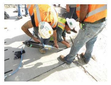
Figure 14.6. Narrow-mouth dowel slot use for repair applications.
