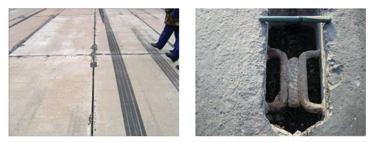
Figure 2.15. Soviet-era precast panels (left) and lifting loops with reinforcing bar (right).
