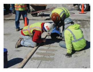
Figure 2.4. Variation of intermittent repair technique with dowel bars installed after panel installation using DBR method.
