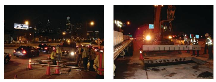
Figure 15.2. Crane placement of panel on four-lane divided highway project.
