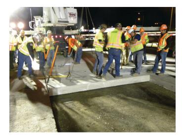
facilities to produce the precast concrete panels. The PCPs are typically overlaid with asphalt concrete (AC) or machine "milled" to correct the profile.
