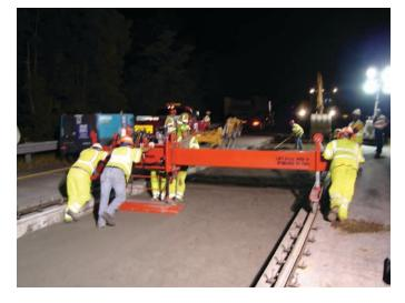
Figure 6.1. Auger-based granular base grading system.
