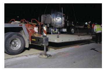
Figure 4.4. Outrigger positioning of lifting crane.
