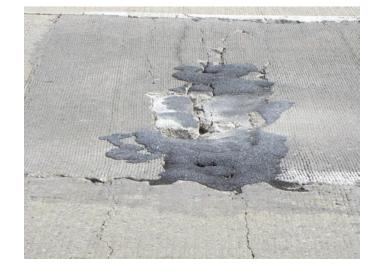
Figure 14.3. Failed FDRs in CRCP.
