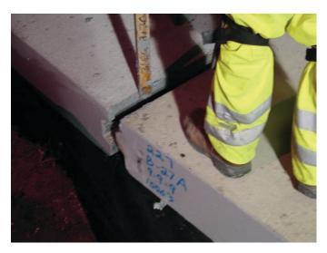
Figure 12.5. Intermediate keyway joint.
