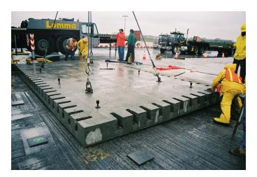
Figure 11.4. Panel placement using setting bolts at New York's LaGuardia International Airport.
