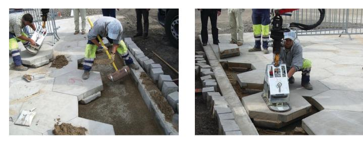
Figure 2.17. Installation of keyed hexagonal panels in France.
