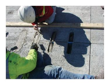
The grout material or the dowel patching material or other repair material can be used to fill the lift insert holes and to repair any surface damage to the panel.
