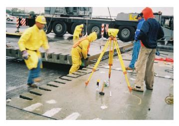
Figure 2.7. An alternate scheme for providing load transfer in JPrCP.
