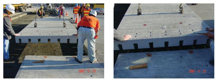
Figure 2.6. A scheme for providing load transfer in JPrCP using dowel slots and embedded dowel bars.
