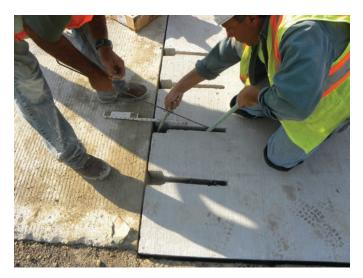
equal the diameter of the dowel bar plus about 0.125 to 0.25 in. (3 to 6 mm) when epoxy is used as the bonding agent.
