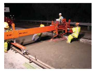
Figure 11.1. Manual base grading.
