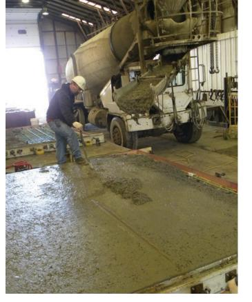
Figure 9.6. Concrete delivery options (transit mixer and bucket).
