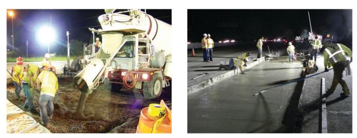
Figure 11.2. Material being directly deposited in PPCP work areas: (left) CTPB placement during Delaware project and (right) LCB placement during California I-680 project.
