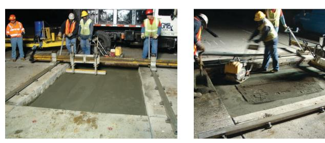
Figure 10.2. Base being graded and compacted within the repair area.
