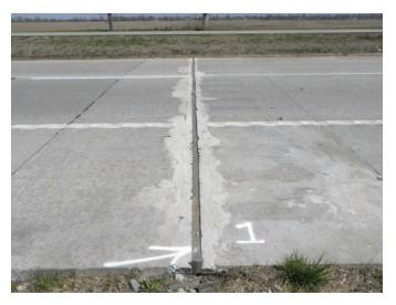
*Figure 3.18. PPCP-reconstructed expansion joint on I-57 in Missouri.*
