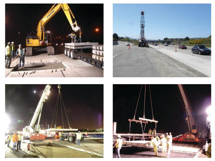
Figure 15.5. Typical panel-lifting equipment.
