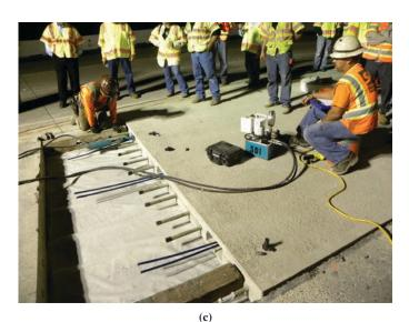
Figure 2.9. Views of the installation of three current versions of PPCP systems with stressing pockets (a) in central panel, (b) at expansion panel, and (c) with posttensioning performed at joint face.
