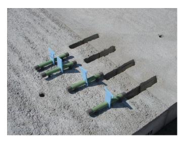
Figure 10.8. Slot patching for DBR.
