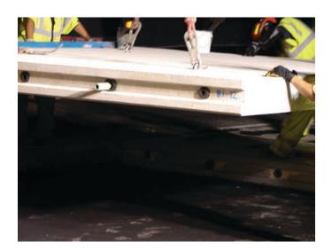
Figure 12.4. Gasket placed on tendon duct.
