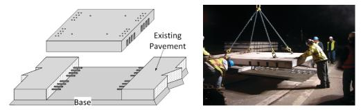
Figure 2.5. Variation of intermittent repair technique with dowel bars positioned in existing concrete pavement.
