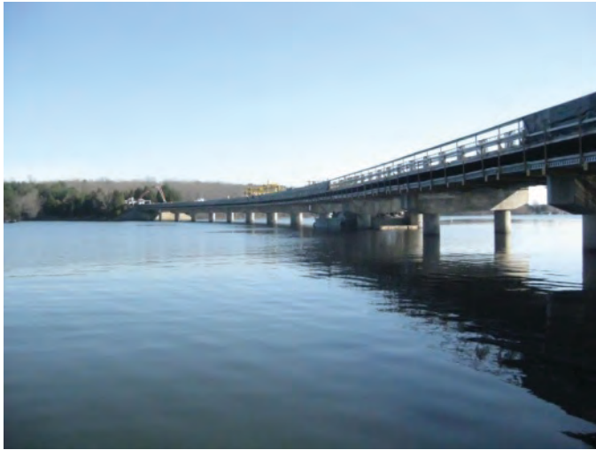
Figure F.1. Route 208 bridge over Lake Anna.
