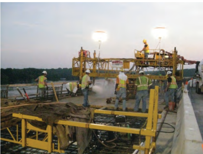
Figure F.7. Water being sprayed on surface.
