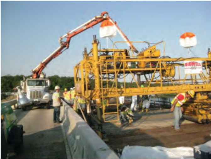
Figure F.5. Pump truck.
