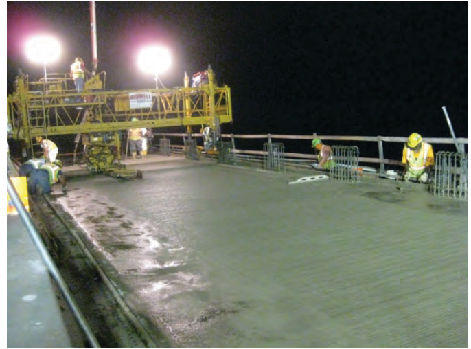
Figure F.8. Hand finishing.
