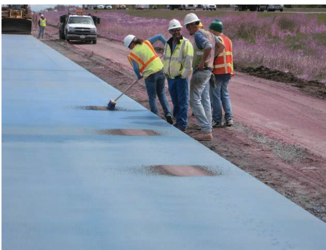
Figure 5.8. Gauging the brushing readiness of the EAC surface with a push broom.
