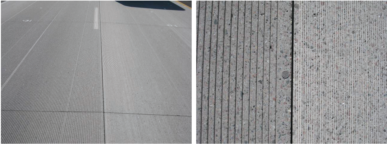
Figure 5.11. Next-generation diamond grinding texture (left lane) and conventional diamond grinding texture (right lane) at MnROAD.
