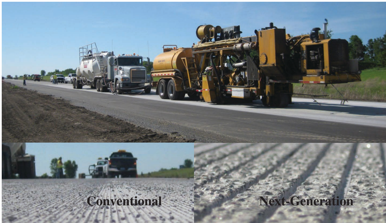
Figure 2.26. The initial learning portion of the EAC texture was diamond ground using conventional grinding in the passing lane and next-generation grinding in the driving lane.
