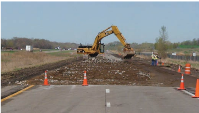
Figure 2.6. Removal of existing concrete pavement for recycling.
