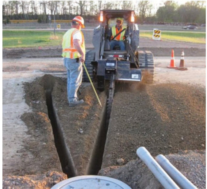
Figure 2.11. Installing conduits to carry and protect the instrumentation cables.
