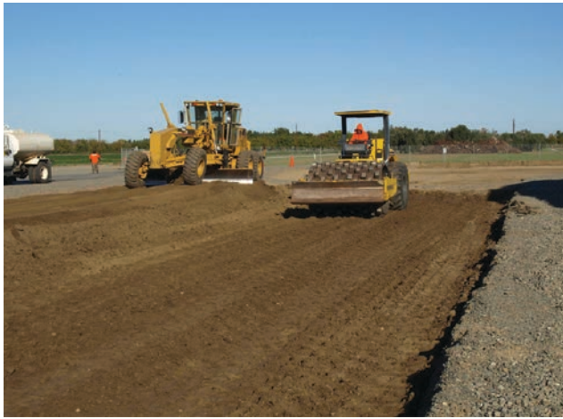
Figure 5.1. Grading and compacting the subgrade and base in preparation for PCC placement.
