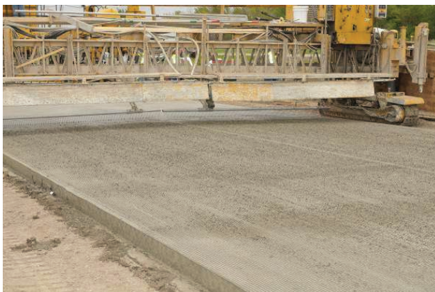
Figure 5.6. Longitudinal tining texture (left) to create adequate surface texture on top of the upper lift PCC and application of curing compound to control surface moisture loss (right).
