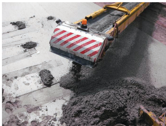
Figure 2.22. Placement of the upper PCC mix on the lower PCC layer.
