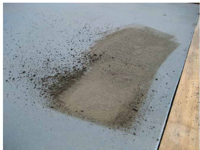
Figure 5.8. Gauging the brushing readiness of the EAC surface with a push broom.
