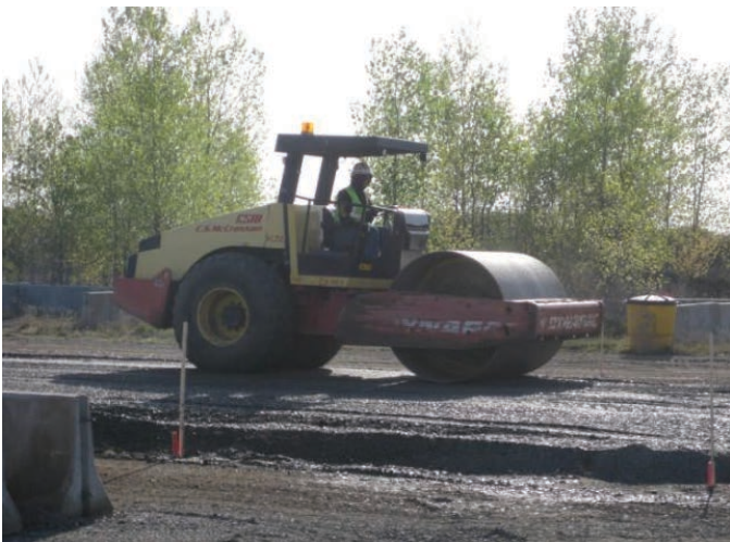
Figure 2.10. Compacting the subbase using a steel drum roller.
