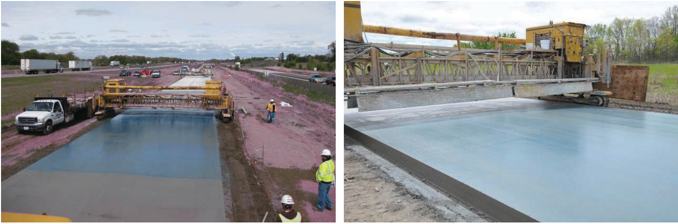
Figure 5.7. Spraying of the curing/retarding compound over the upper PCC at MnROAD.
