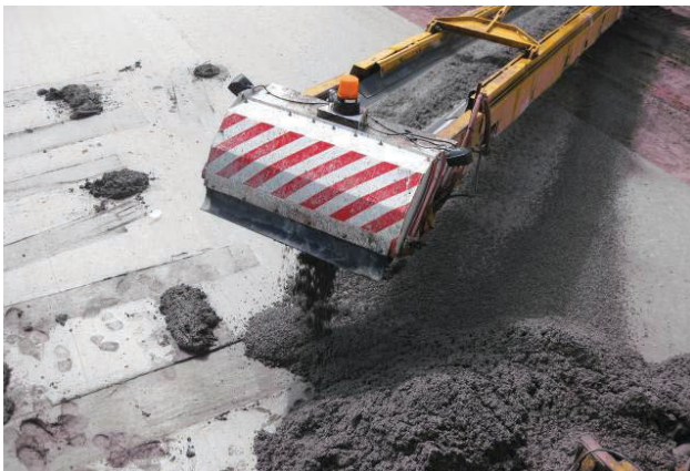
Figure 5.4. Paving the upper PCC layer.
