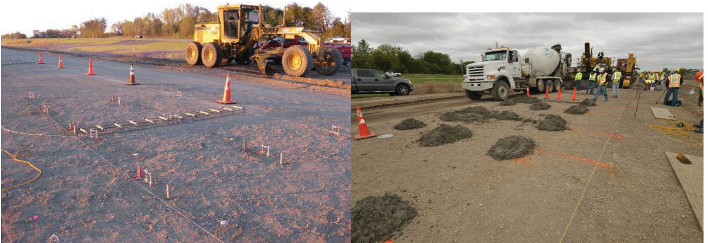
Figure 2.14. Overview of instrumentation packed in concrete before PCC paving.
