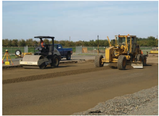
Figure 5.1. Grading and compacting the subgrade and base in preparation for PCC placement.
