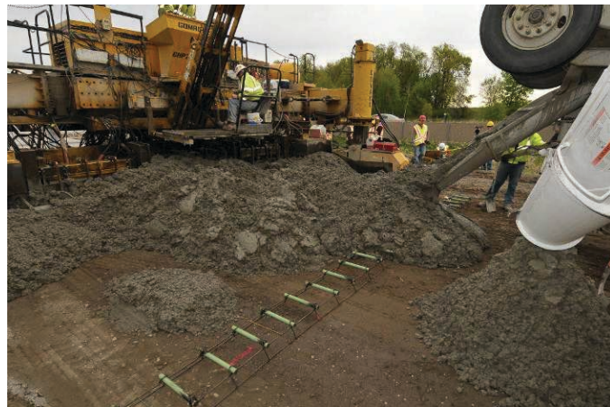
Figure 2.21. Placement of the lower PCC mix.
