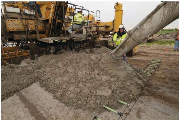
Figure 5.2. Paving the lower PCC layer.
