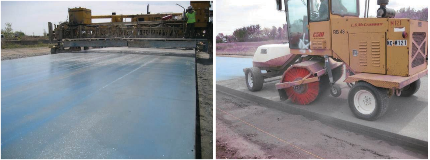
Figure 2.23. Treated surface and finishing platform (left). Equipment for EAC brushing (right).
