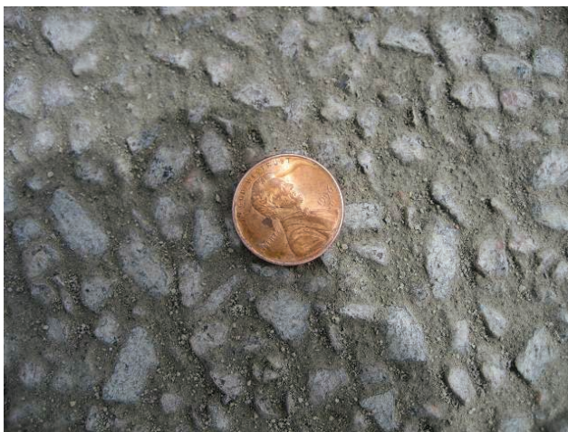
Figure 5.10. Properly brushed EAC surface.
