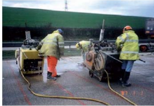
Figure 7. Sawing of concrete slabs. (Jordan et al. 2008)
