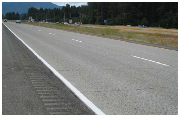
Figure ES.1. Photo of 35 year old unbonded PCC overlay on I-90.
