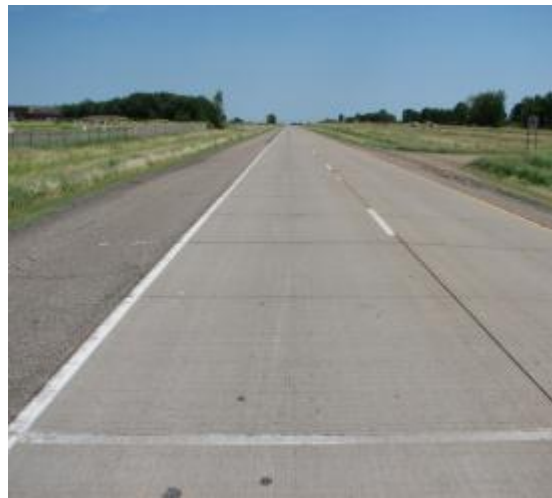
MnRoad Cell 92. Bonded concrete overlay 6 in. thick with a 10 ft by 12 ft spacing with dowels. Performance: Longitudinal cracking in some panels but no faulting. Replaced in 2010.
