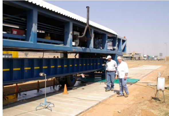
HVS testing of 50 mm thin CRCP
