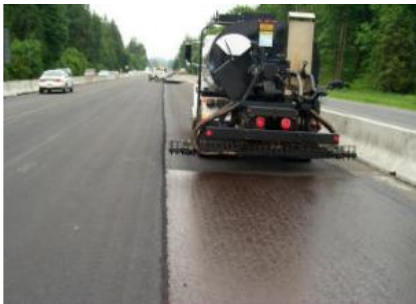
(a) Good tack coat
