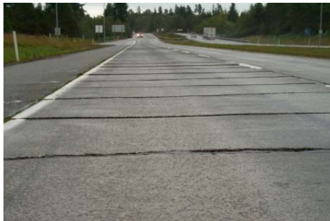
Average Fault ~ 0.25 to 0.5 in. (Source: Pavement Interactive)
