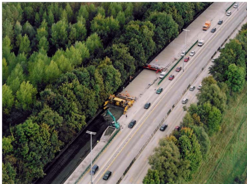
Figure A.22. CRC overlay construction on E40/A10 in Belgium. (Photo: Hall 2007)
