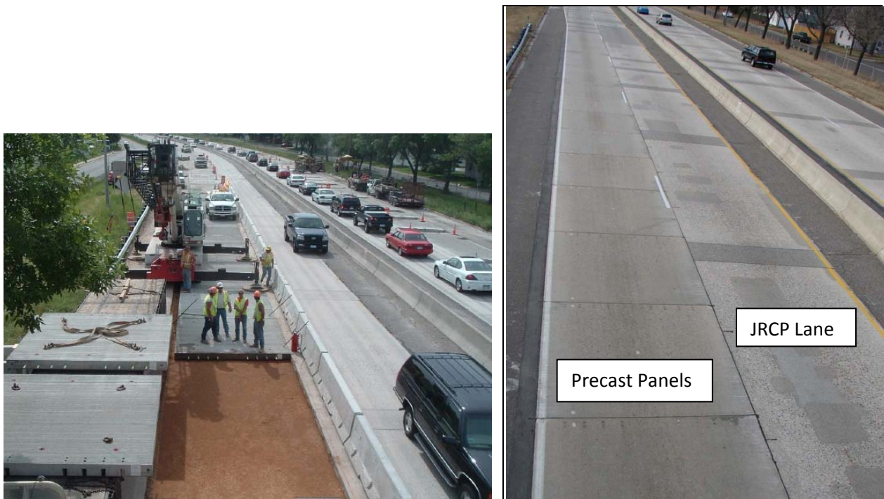
Figure 5. Precast Section—Minnesota TH 62. (Photos from Burnham, 2007)
