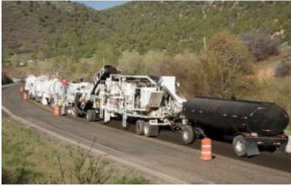
(a) CIPR Train with engineered asphalt emulsion
