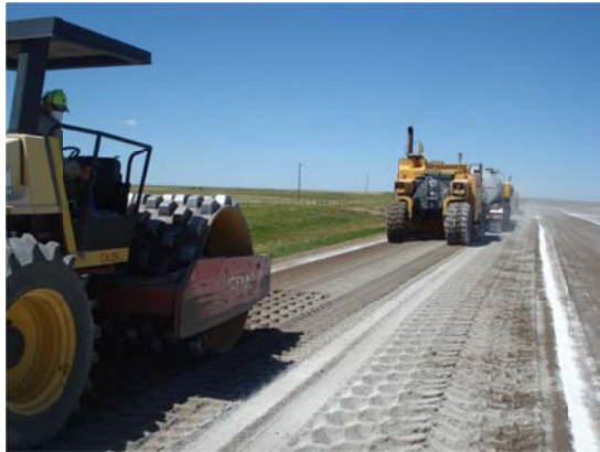
(c) FDR with asphalt emulsion and dry lime
