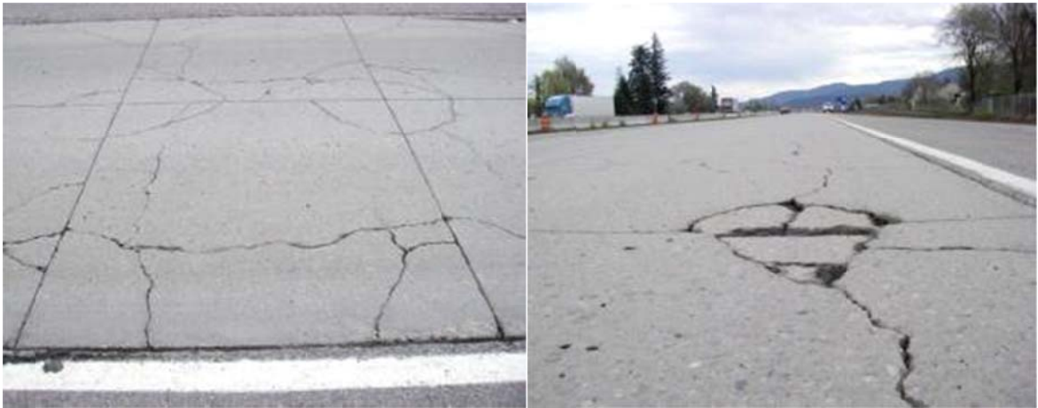
3 in. Bonded PCC overlay of HMA following 8 years of service.
