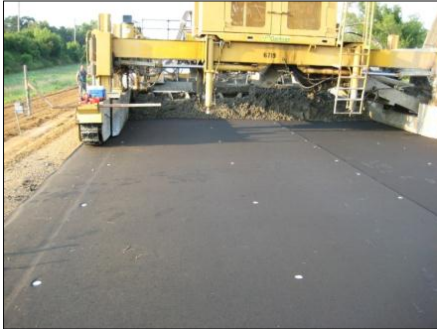
Figure 25. Placement of non-woven fabric as an interlayer. (From Tayabji et al [2009])
