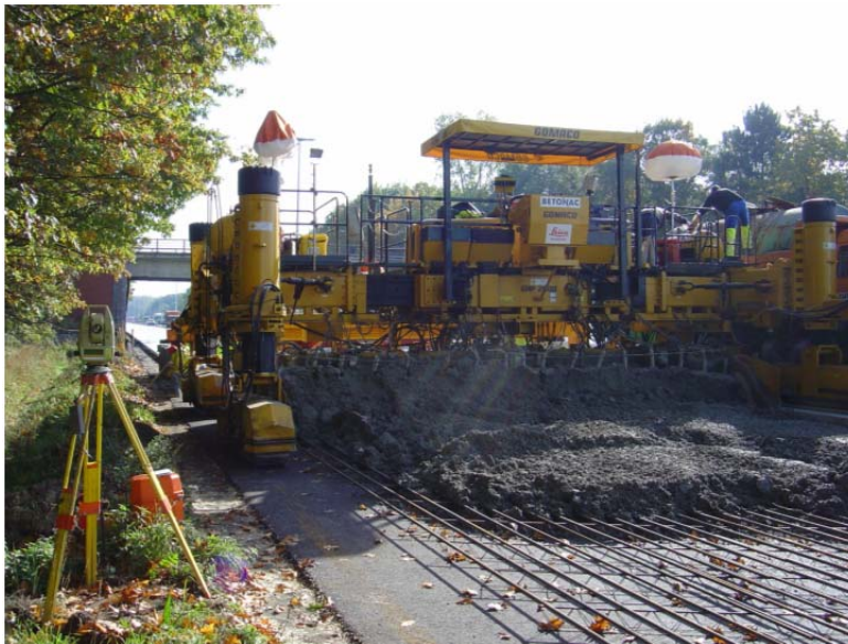
Figure A.23. CRC overlay paving on E40/A10 in Belgium. (Photo: Hall 2007)
