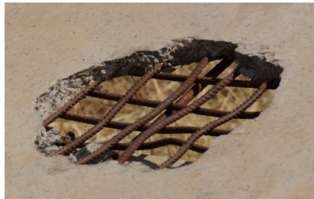
Close-up of reinforcing.
