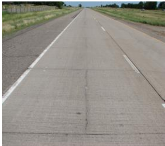
MnRoad Cell 92. Bonded concrete overlay 6 in. thick with a 10 ft by 12 ft spacing with dowels. Performance: Longitudinal cracking in some panels but no faulting. Replaced in 2010.
