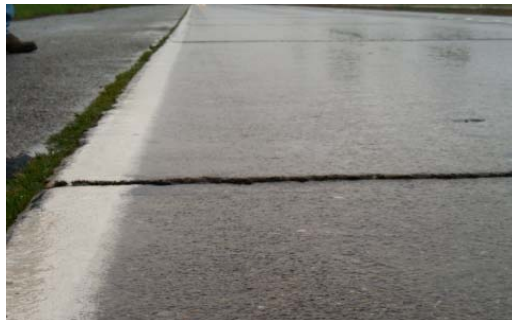
Average Fault ~ 0.5 in. (Source: Pavement Interactive)
