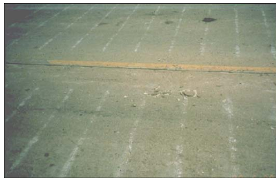
(b) Fractured Slab with Guillotine Hammer
