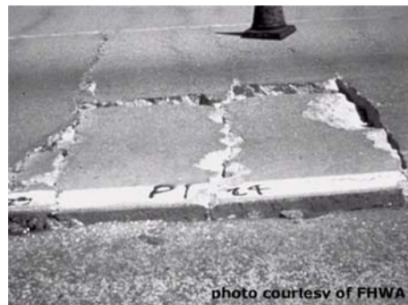
Advanced Stage for a Punch-out (Source: FHWA)
