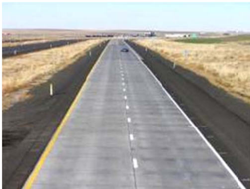
JPCP constructed on HMA base
