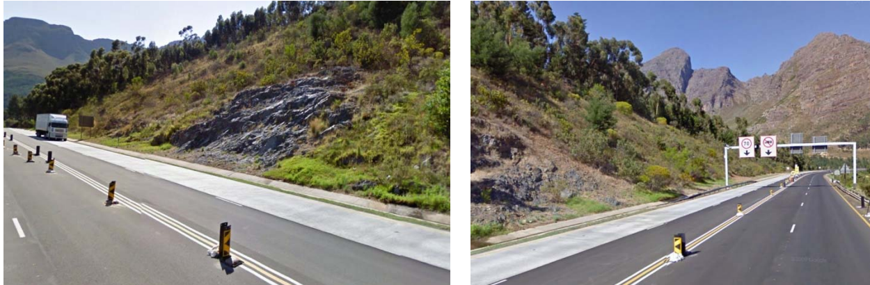
Figure 2. UTCRCP on the N1 Highway near Cape Town. (Photos: Wynand Steyn)
