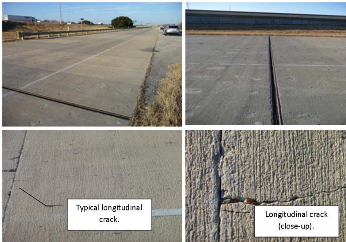
Figure 4. PPCP Section—Texas I-35 Frontage Road—Photos December 2010. (Photos: Joe Mahoney)
