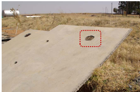
Previously tested section illustrating reinforcing.
