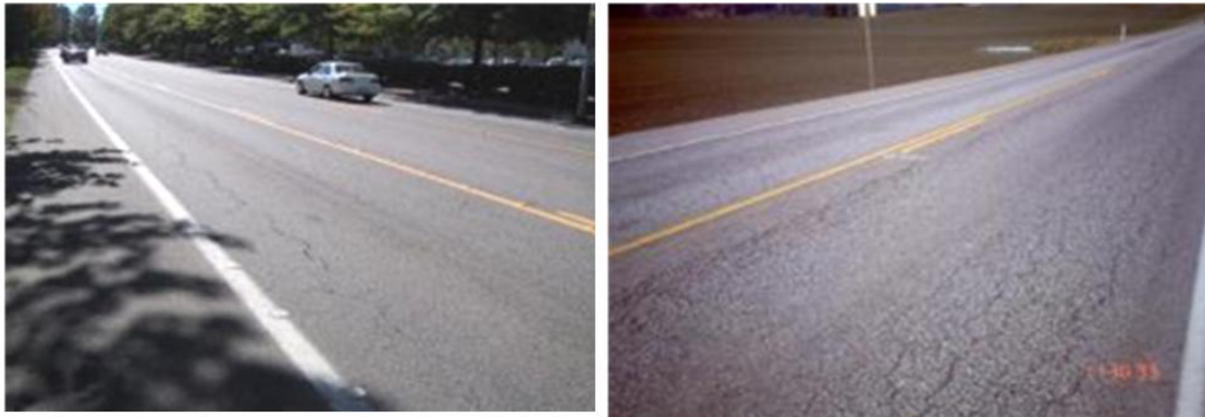
Figure 28. Illustrations of top-down cracking in Washington State. (the upper photos are from Interstate 90; the bottom photos local streets in western Washington)
