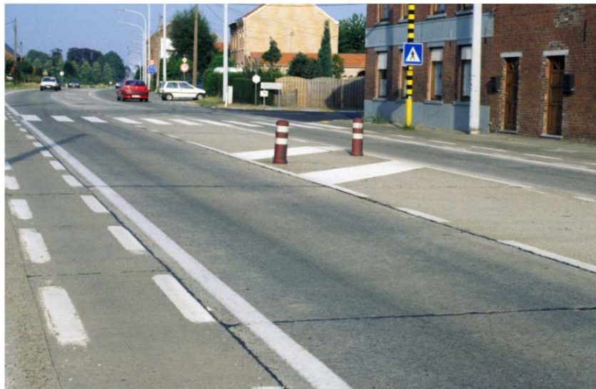
Figure A.21. Belgium's first concrete overlay after 45 years in service.
