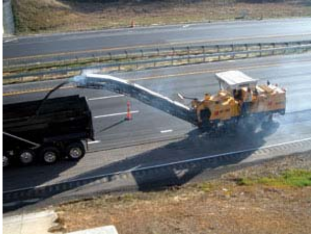
Figure 1. Typical milling operation of existing HMA layer. (WSDOT, 2010)
