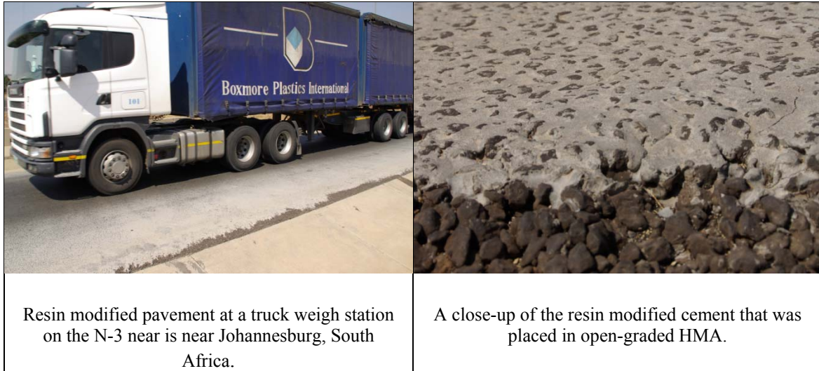
Figure 3.10. Resin modified pavement in South Africa.(Photos: Joe Mahoney)
