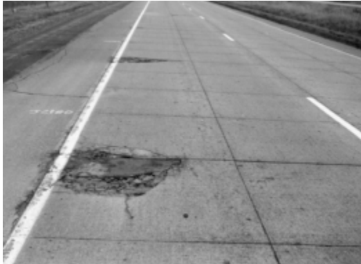
MnRoad Cell 95. Bonded concrete overlay 3 in. thick with a 5 ft by 6 ft joint spacing in November 2003.
