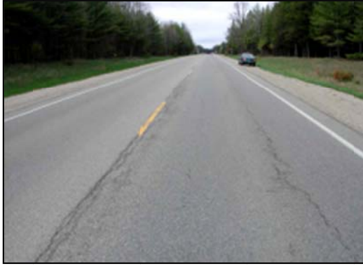
Figure 30. Two views of longitudinal top-down cracking in Michigan. (the photo on the right is HMA placed over rubblized PCC pavement)
