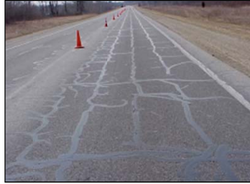
Figure 30. Two views of longitudinal top-down cracking in Michigan. (the photo on the right is HMA placed over rubblized PCC pavement)
