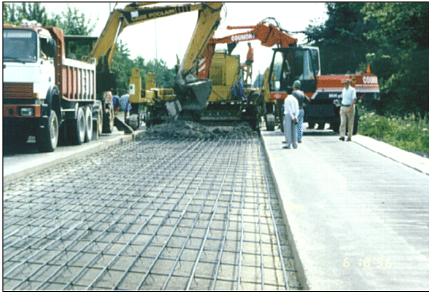
Figure A.26. CRC inlay construction in Belgium. (Photo: Hall 2007)
