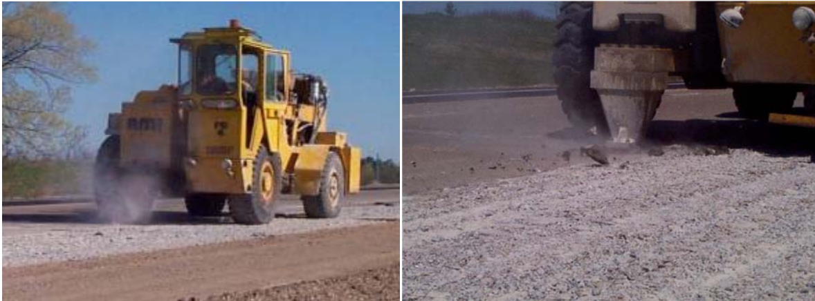
(a) Resonant breaker machine
