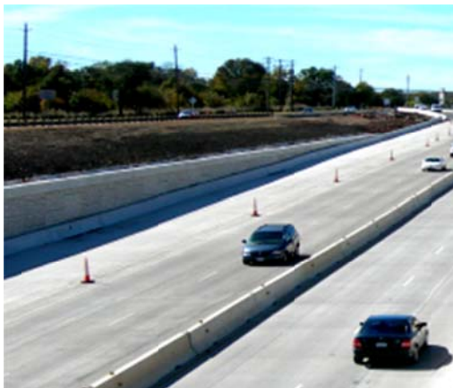
CRCP Constructed on HMA Base
