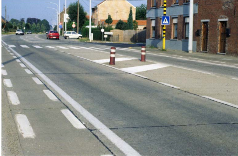
Figure 3.4. Belgium’s first concrete overlay after 45 years in service. (Photo: Hall 2007)
