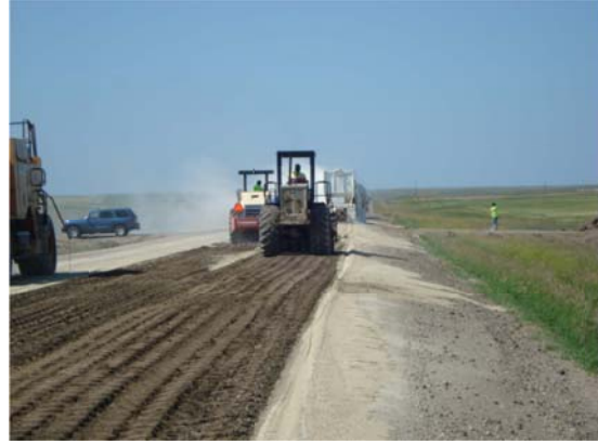
(b) FDR with cement/fly ash stabilizer
