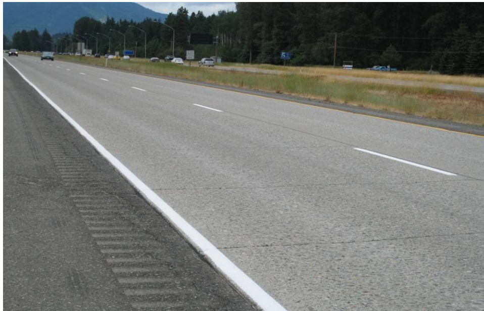
Figure 3.3. Photo of 35 year old unbonded PCC overlay on I-90 MP 74.
