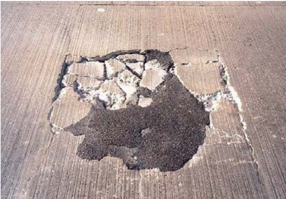
(b) Severe punchout block
