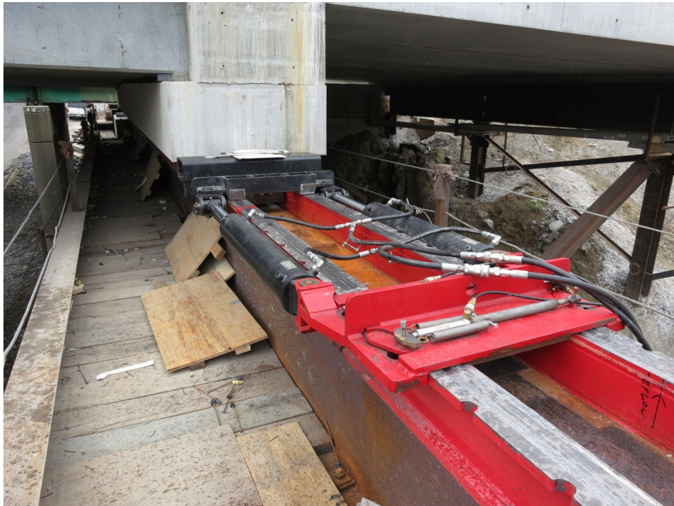
Figure 2. Slide track and push/pull jacks—I-84 bridge lateral slide, New York.
