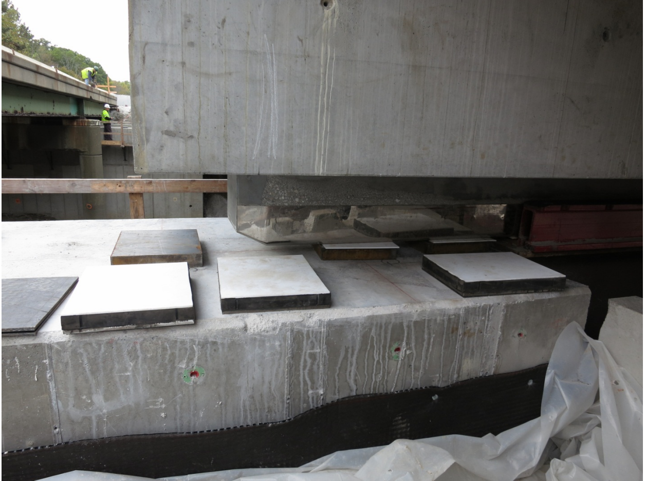
Figure 5. PTFE slide pads on elastomeric bearings—I-84 bridge lateral slide, New York.
