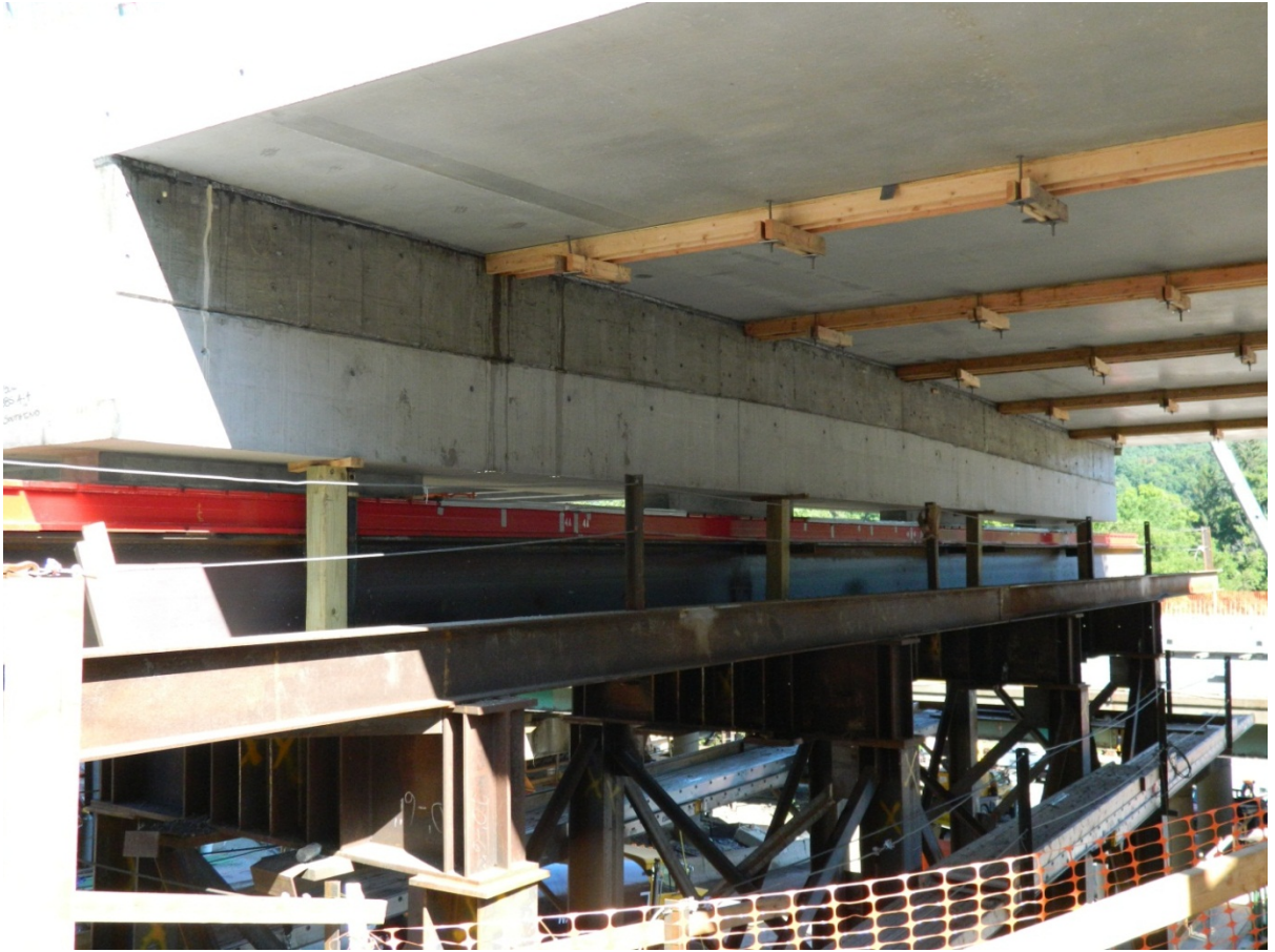
Figure 4. End diaphragm with slide shoes—I-84 bridge lateral slide, New York.
