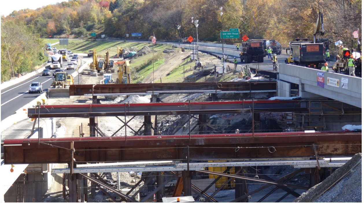
Figure 1. Temporary supports and slide tracks—I-84 bridge lateral slide, New York.
