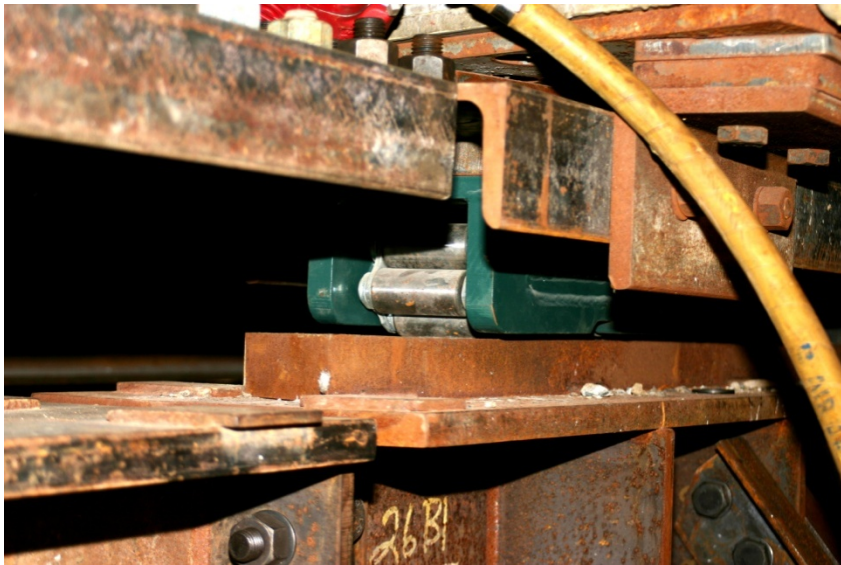
Figure 3. Roller bearing–Hillside Avenue bridge roll-in, New York.
