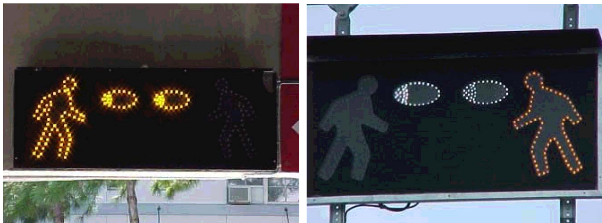
Figure 3, Garage and crosswalk signals
