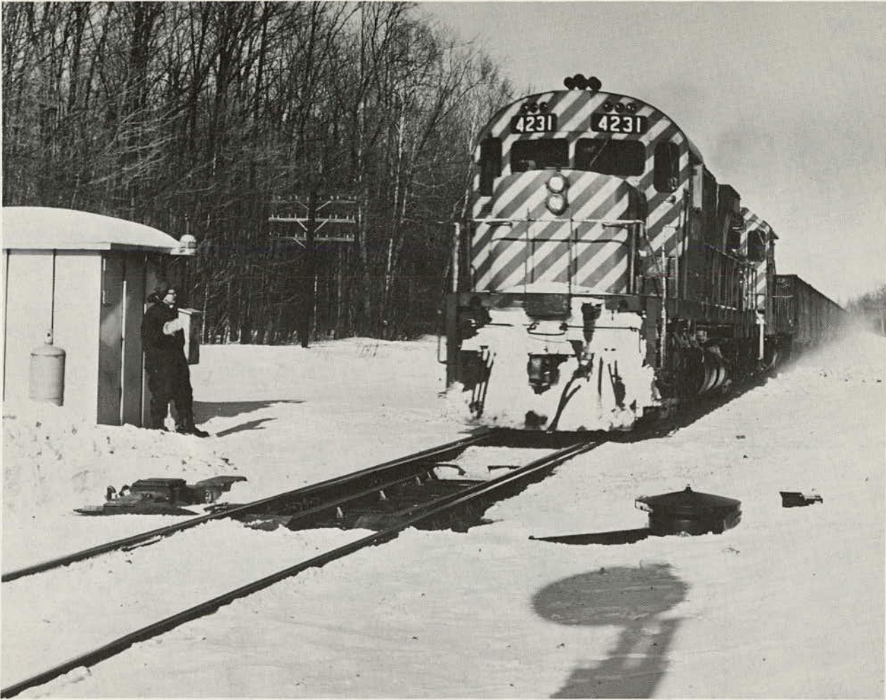
Figure 2. Pulse jet switch heater at Perth, Ontario.
