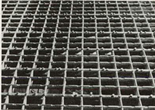
Fig. 14 Overall view of open steel grid bridge decks
