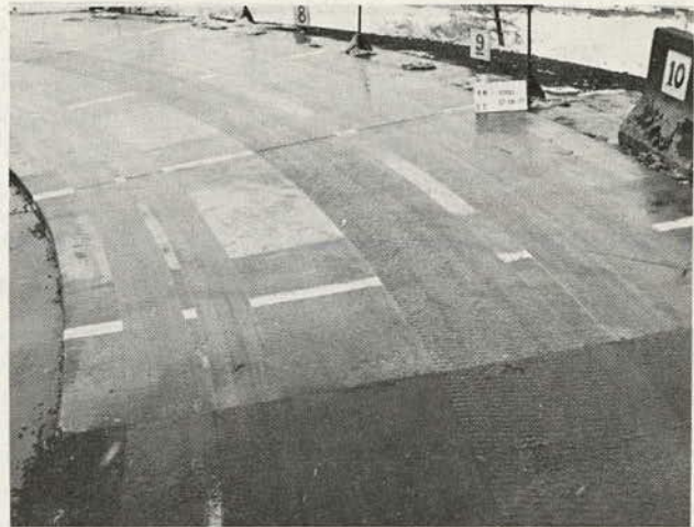
Figure 6. Portland Cement Concrete After Formula Application
