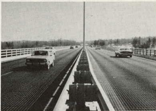
Fig. 14 Overall view of open steel grid bridge decks
