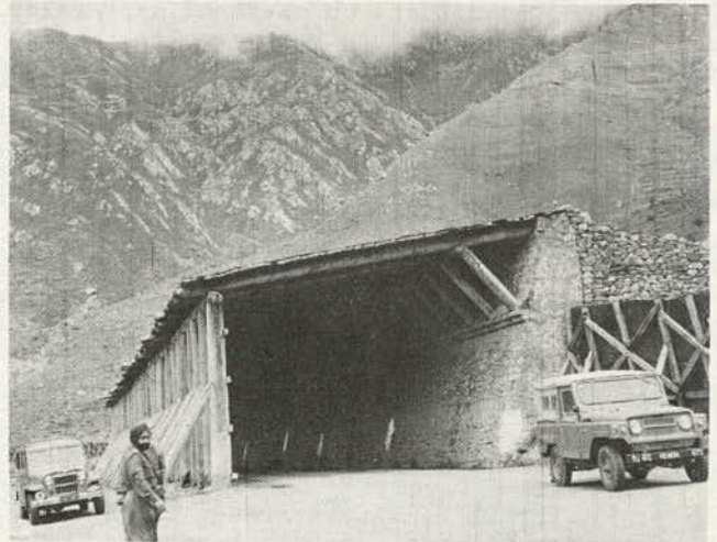
Photo 4. A typical snow-shed - one of the few protective structures provided for safe & unhindered movement of traffic.
