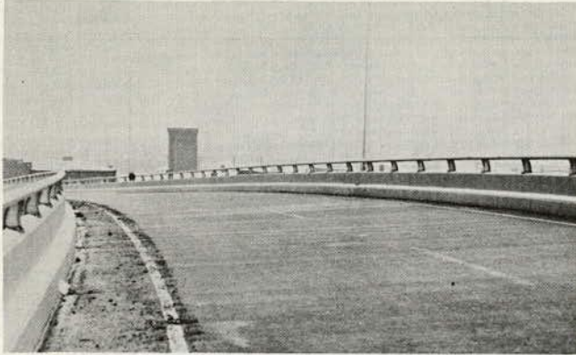
Figure 15. Heated Pavement (January 14, 1977).
