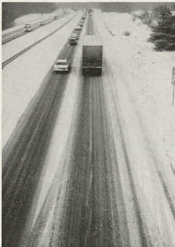
Fig. 10 Pavement prior to brine application
