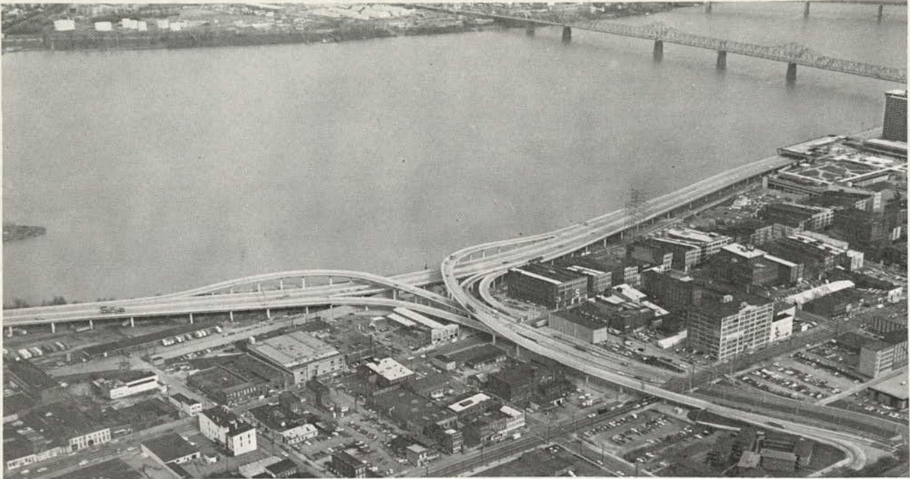
Figure 11. 9th-Street Interchange, Looking toward River.
