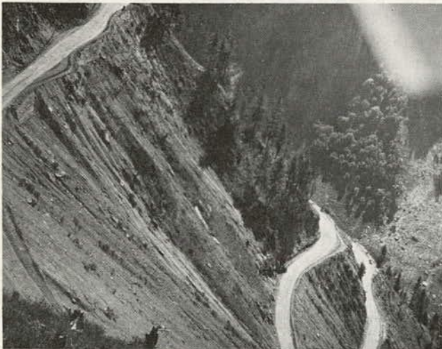
Photo 3. Road winding around a steep hill slope.
