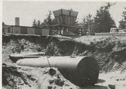
Fig. 7 Tanks used to store brine with brine-making unit in background
