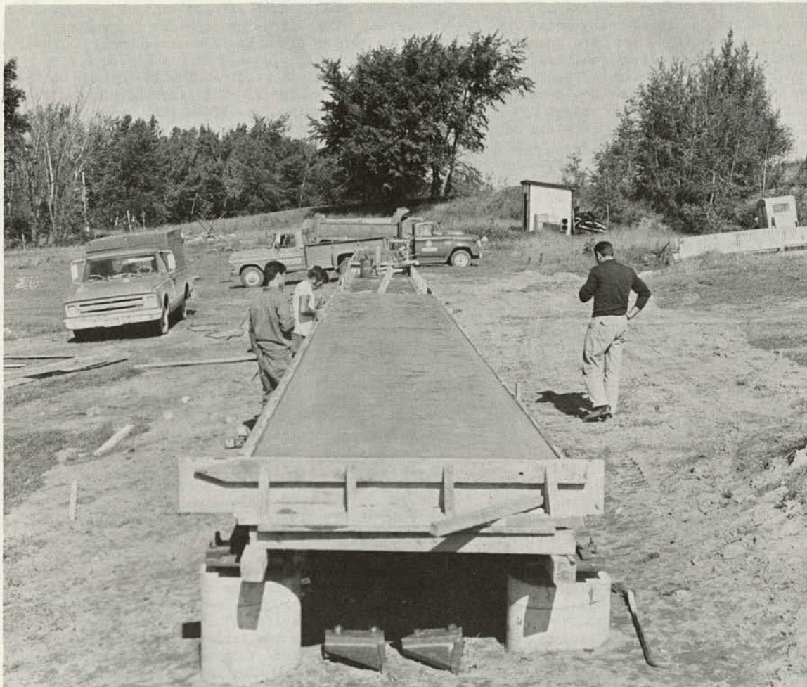
Figure 1. Experimental track under construction.
