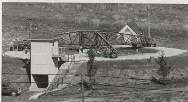
Figure 1. A View of the Present G.A. Riedesel Pavement Testing Facility
