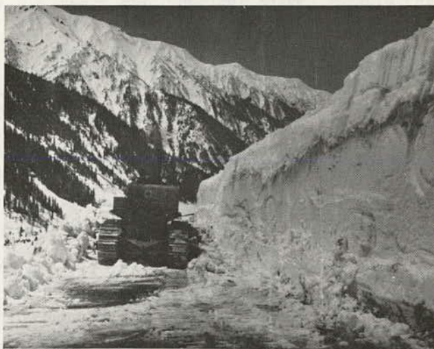
Photo 9. Snow clearance in progress.
