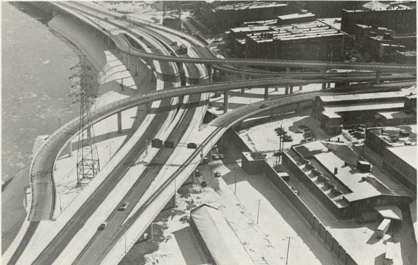
Figure 17. Aerial View of the 9th-Street Interchange on February 2, 1978, Showing the Distinct Difference between Heated and Non-Heated Sections.
