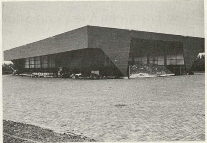
Figure 1. Covered salt store (the Netherlands).
