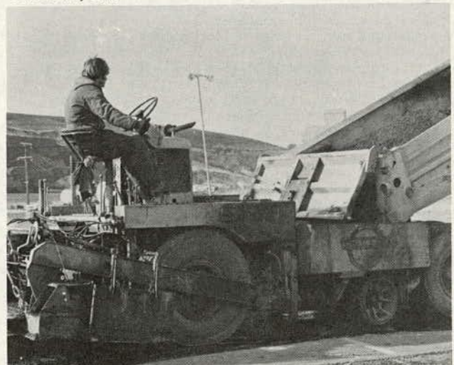
Figure 3. Placement of Asphalt, Sections 21-23, October 27, 1976
