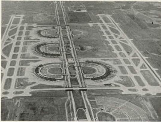
FIGURE 1 D/FW AIRPORT AT DALLAS/FORT WORTH, TEXAS
